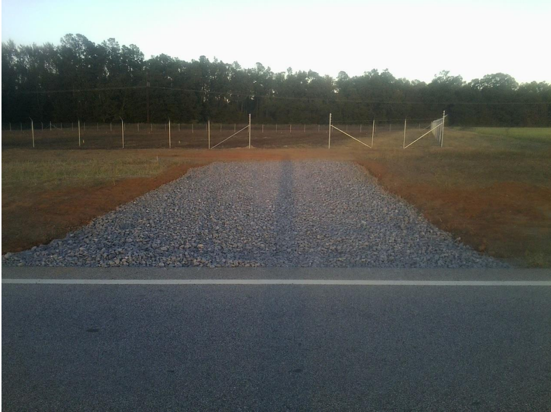
Picture 12 – Stabilized Construction Entrance
