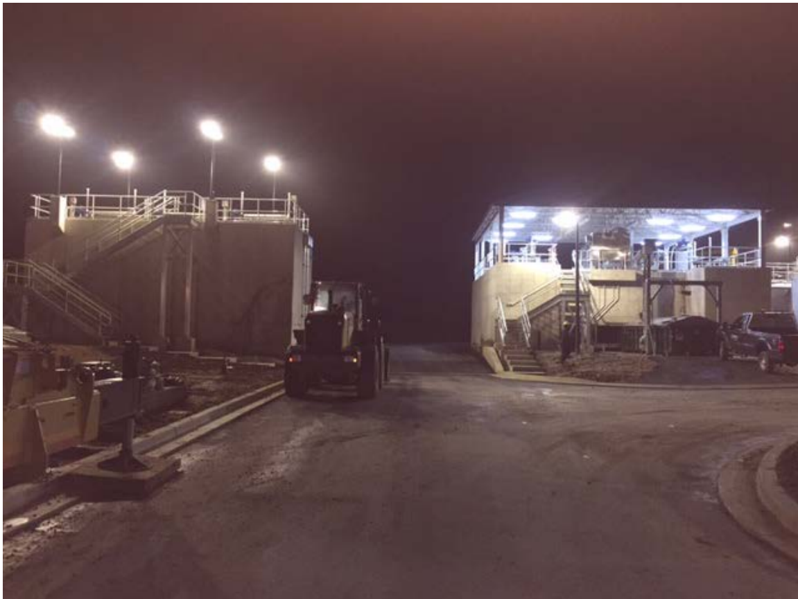
Headworks Facility at night (Distribution Structure on left and Screen Building on right)
