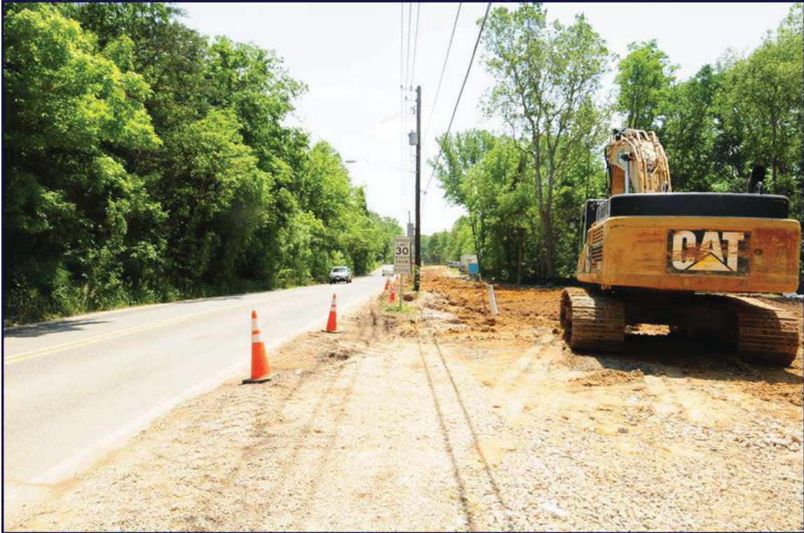
Pipe installation along Livingston Road
