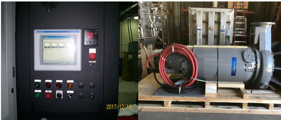
New Variable Frequency Drives (3 VFDs)
