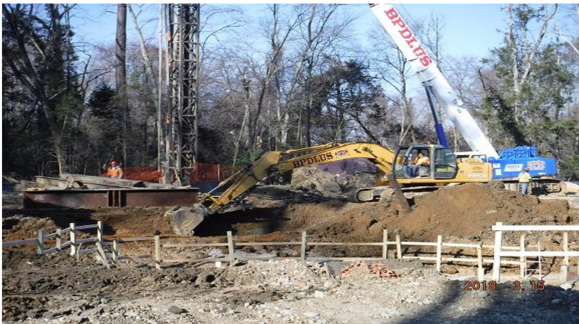
Excavation for valve vaults at pumping station
