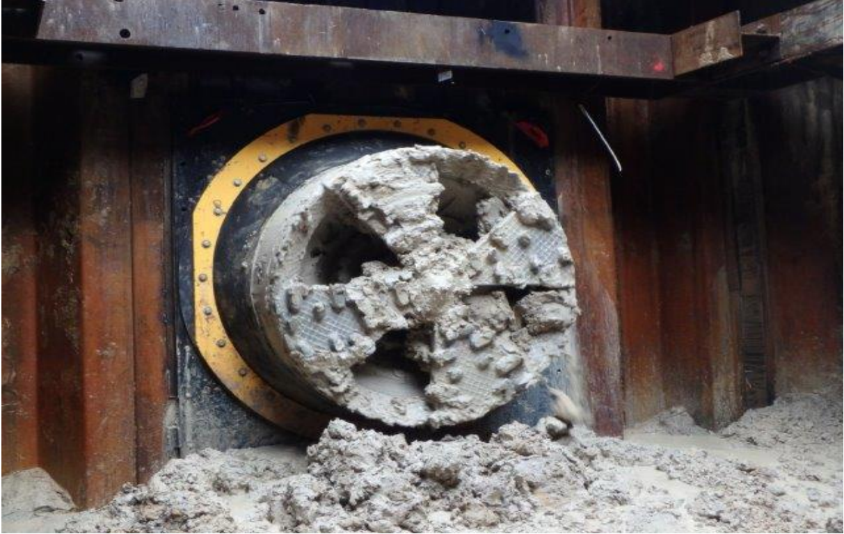
Hole Thru on recent tunnel crossing Swan Creek Road
