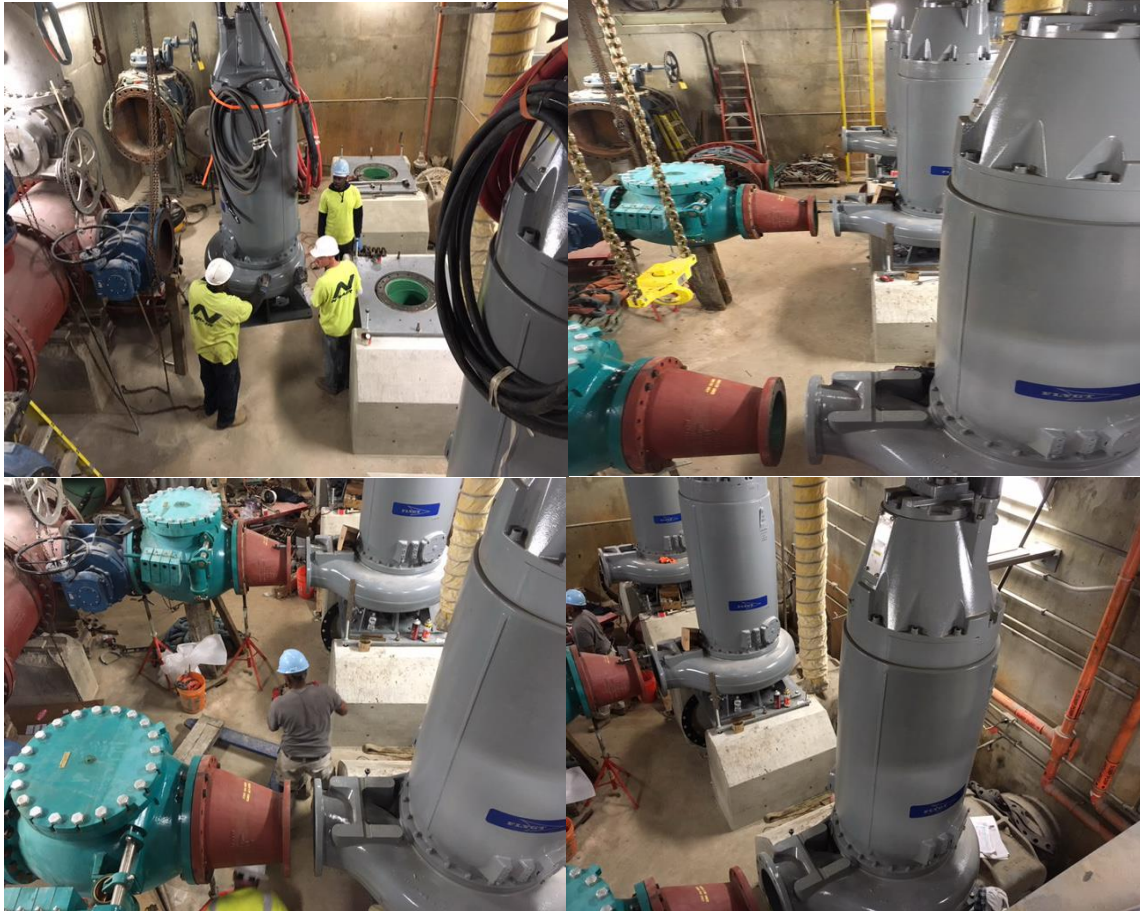
Installation of pumps
