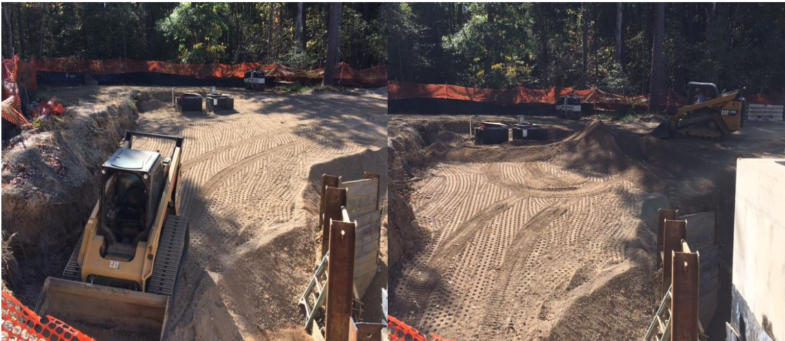
Backfilling operations at the pumping station
