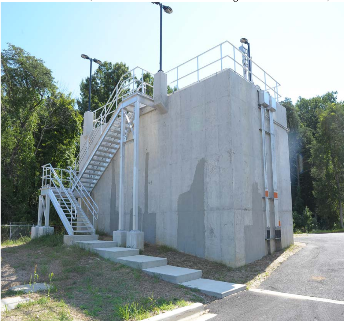
Influent Distribution Structure
