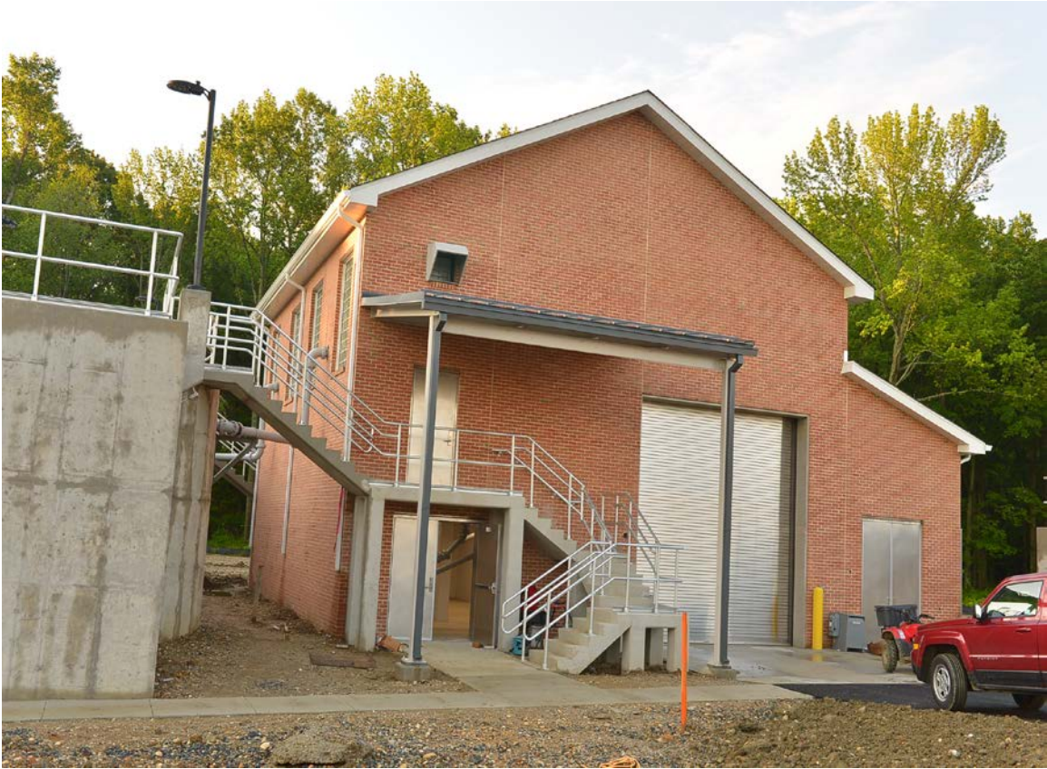
Grit Building and Electrical Room
