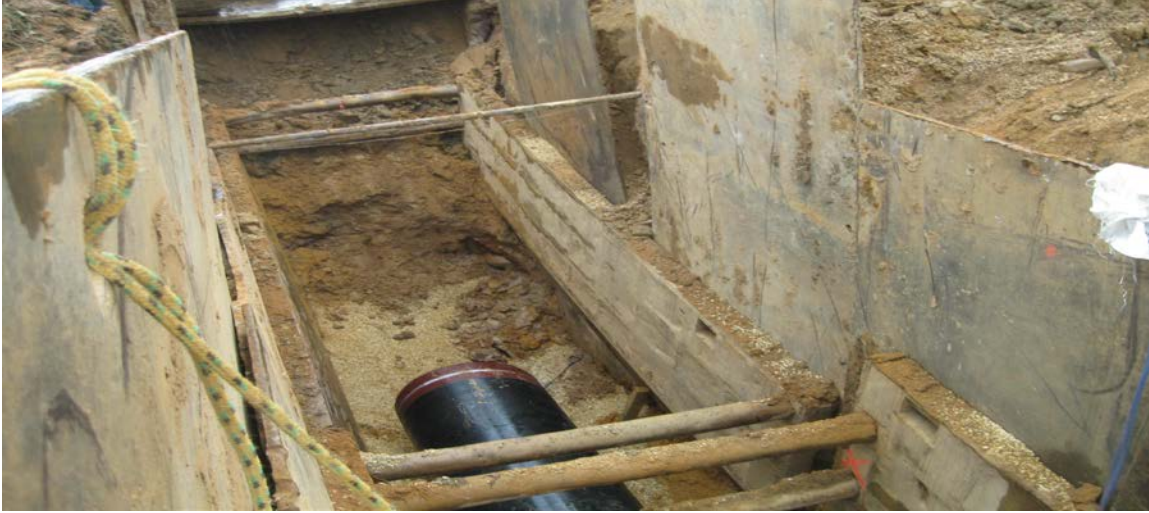
Installation of 48" Force Main along MD 210
