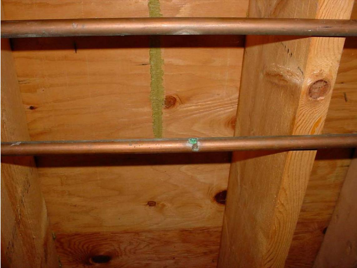
*Figure 1: Pipe with Pinhole Leak (Courtesy of WSSC)*
