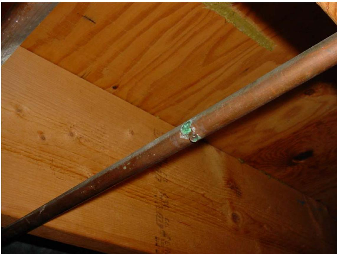
*Figure 2: Shows Further Details of Pinhole Leak (Courtesy of WSSC)*
