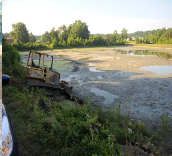
Clearing and dewatering for Storage Facility
