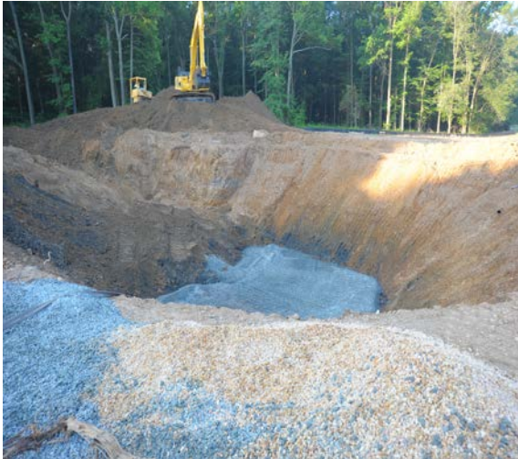
Foundation for New Grit Building
