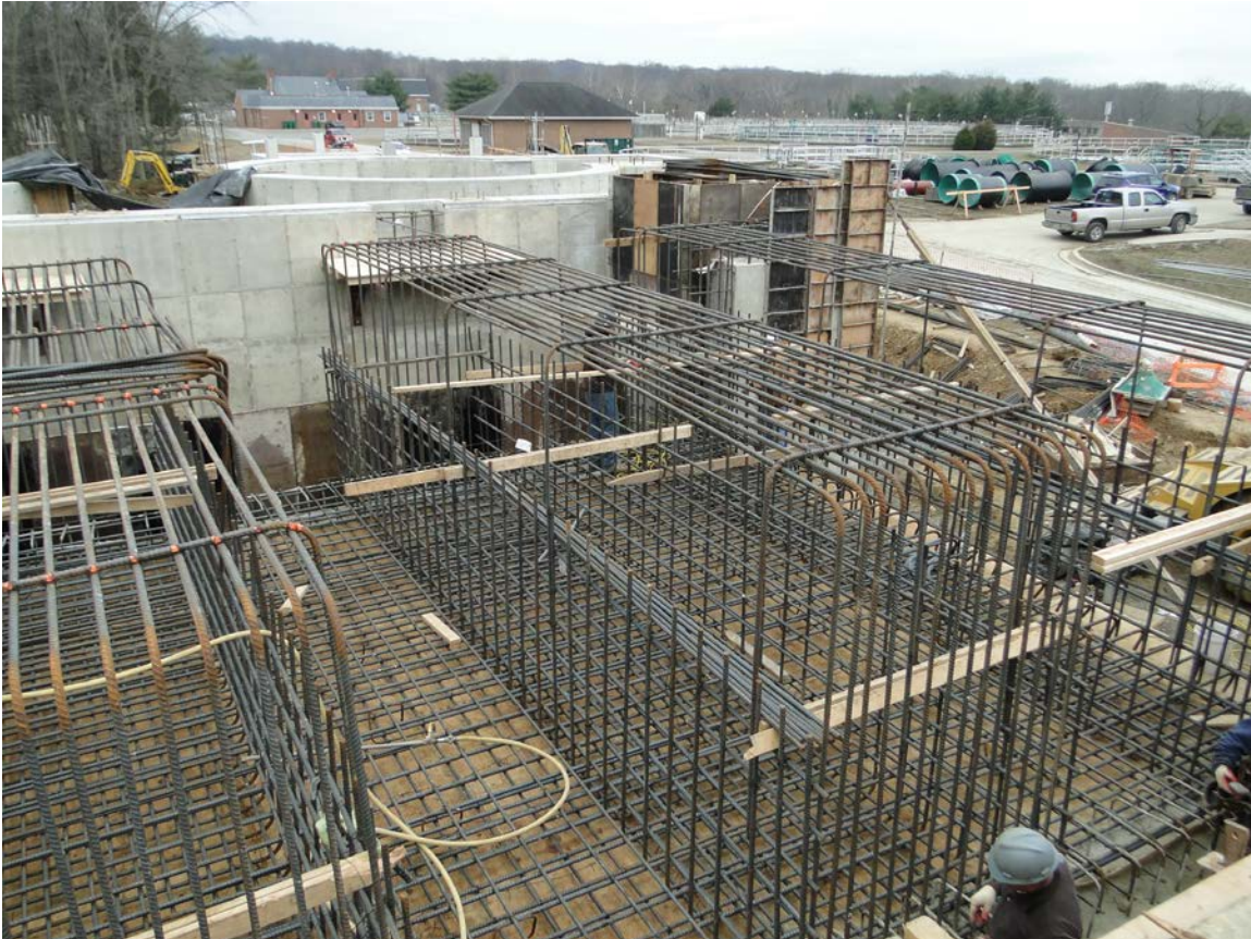
Headworks Facility Construction
