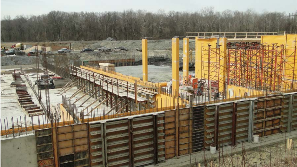
Storage Facility Construction – Base slab and walls
