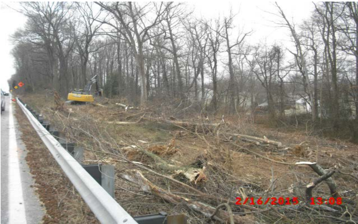
Tree clearing for pipeline along MD 210 - south of Swan Creek Road
