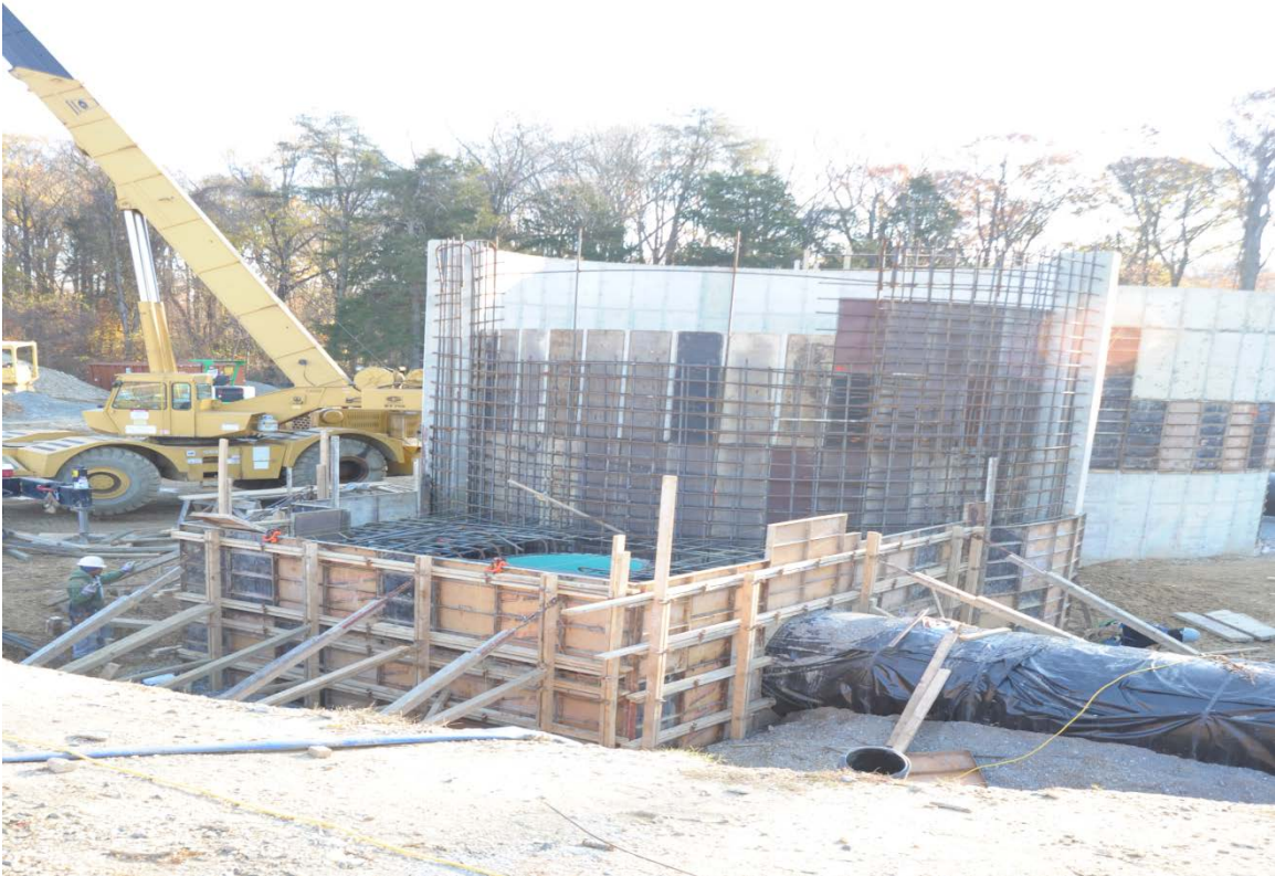
Headworks Facility Construction
