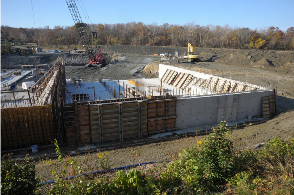
Storage Facility Construction – Base slab and walls
