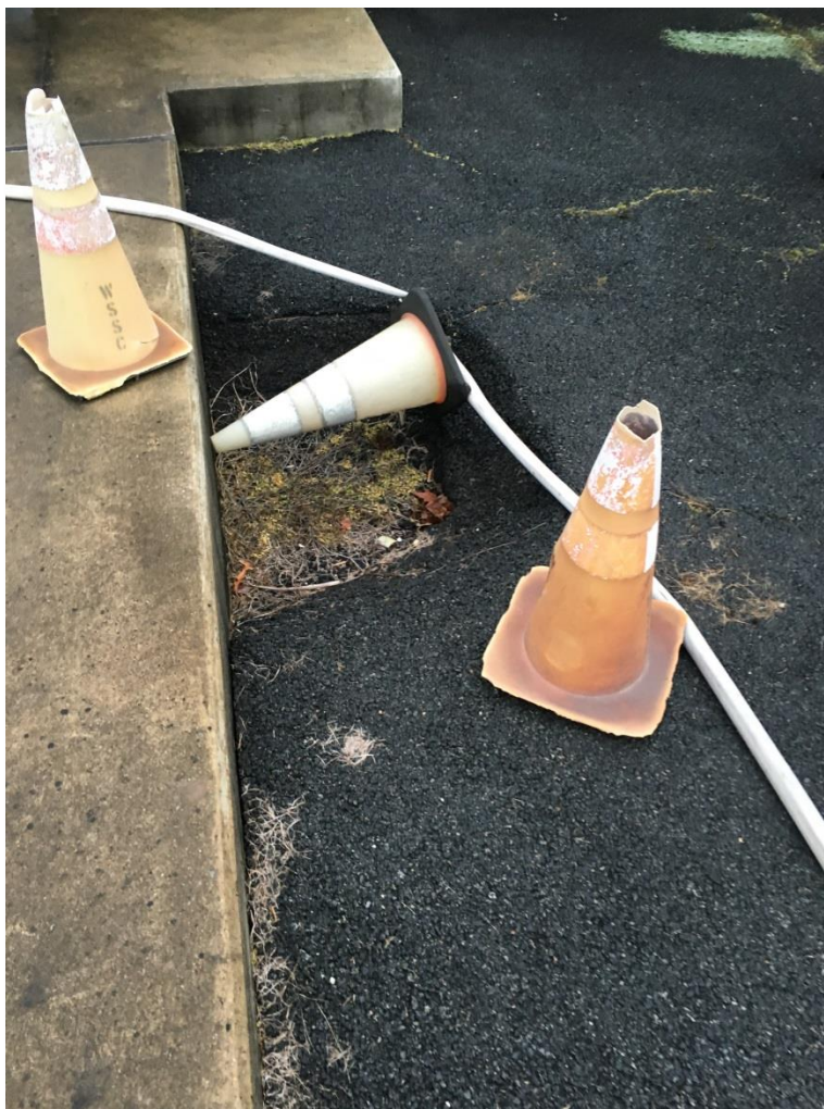
Figure WW.10 Improper Delineation of a Tripping Hazard Shown at Piscataway
