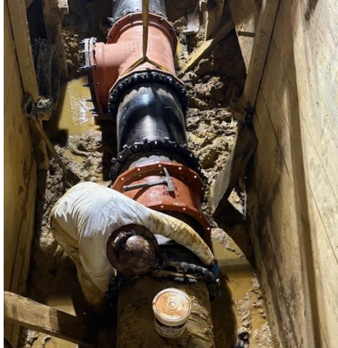
Pictured above: 20-inch water main installation on New Hampshire Avenue, September 2026
