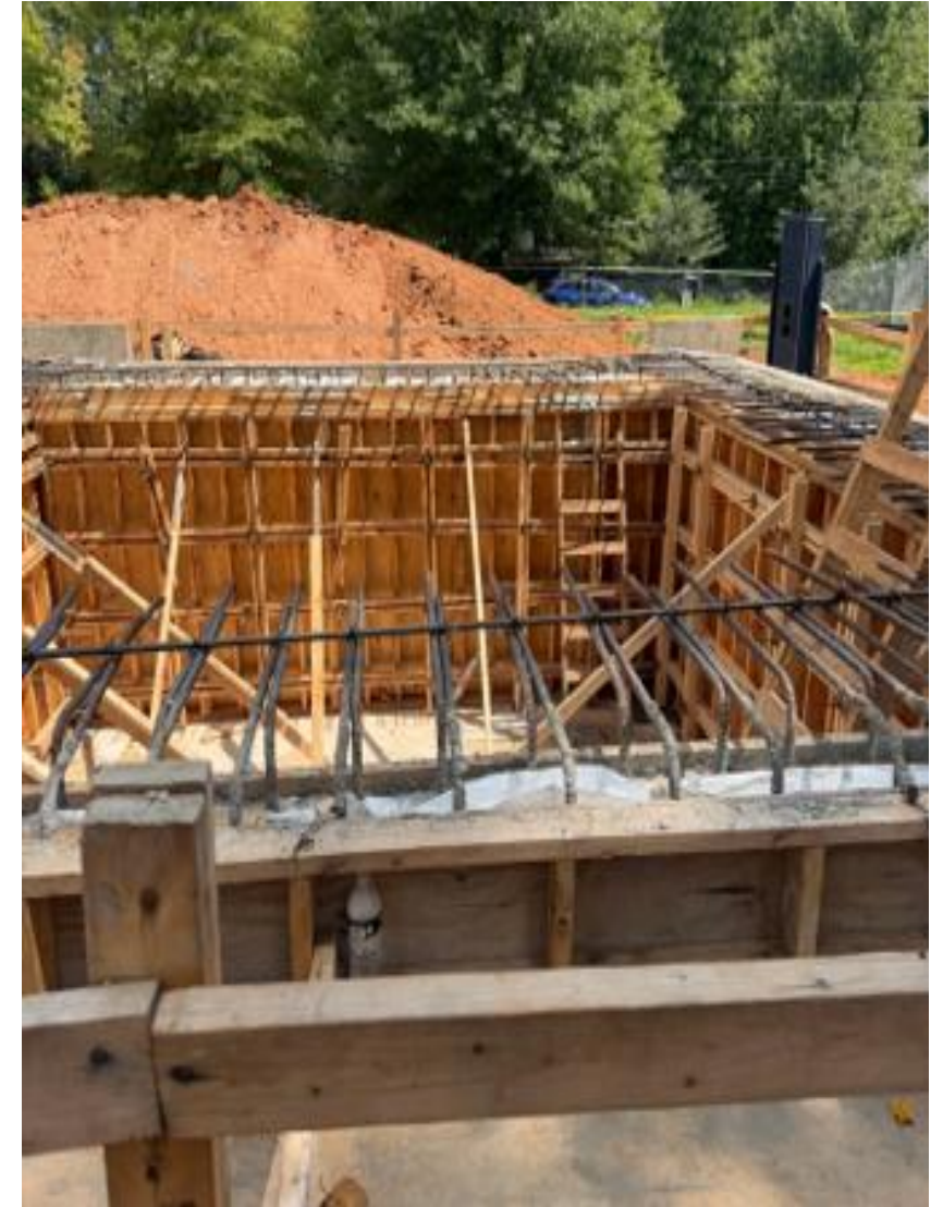
Altitude valve vault under construction
