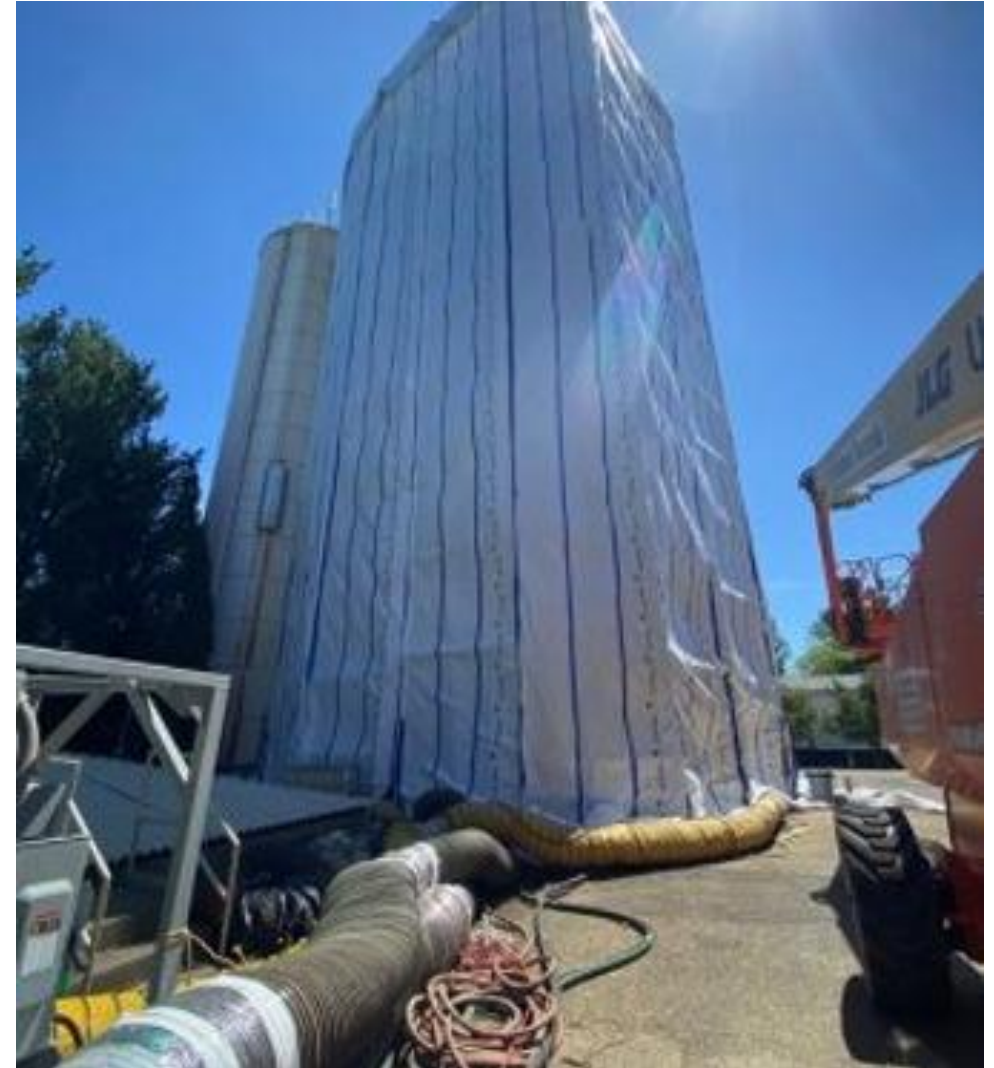
Scaffold type class 2-A containment system
