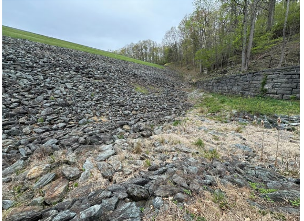
Bottom of little Seneca Dam, looking up
