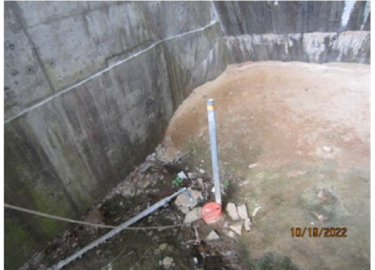
view of Brighton Dam piezometer b-6
