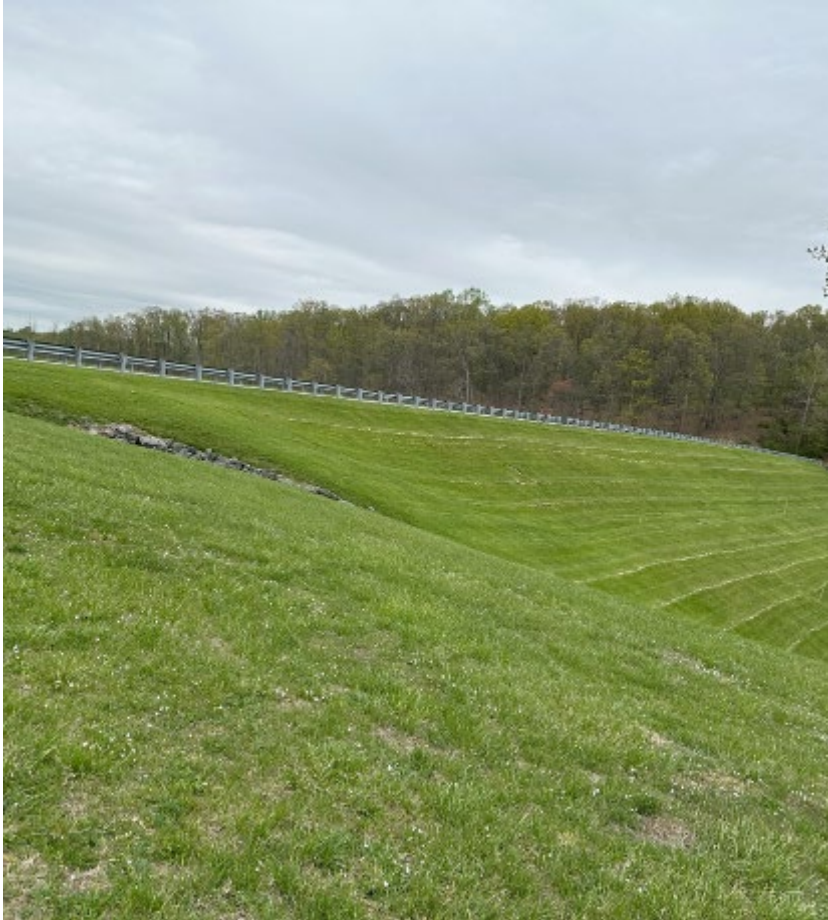
South end of little Seneca Dam, looking north
