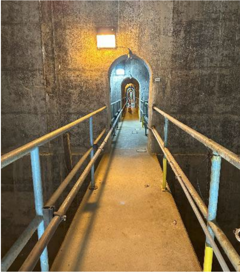
view of Brighton Dam catwalk, looking north-east
