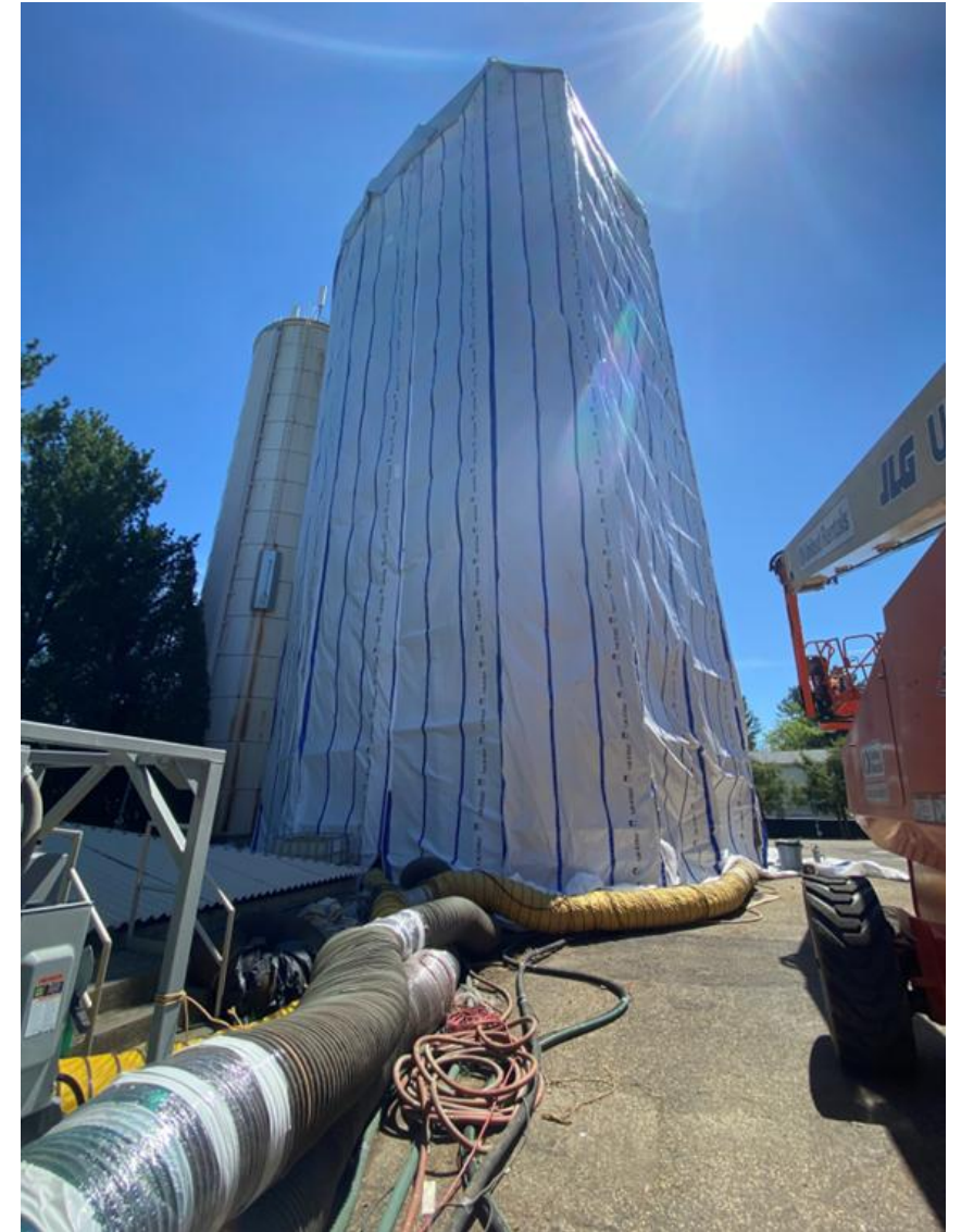
Example of a containment system
