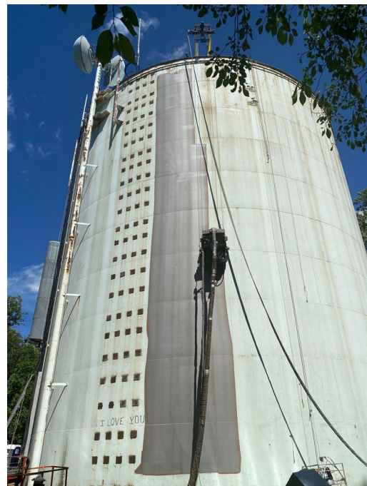
Faster Blaster equipment operating on the tank exterior.
