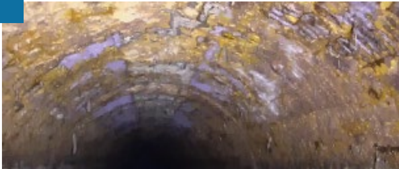
102" Anacostia Sewer Main Corrosion
