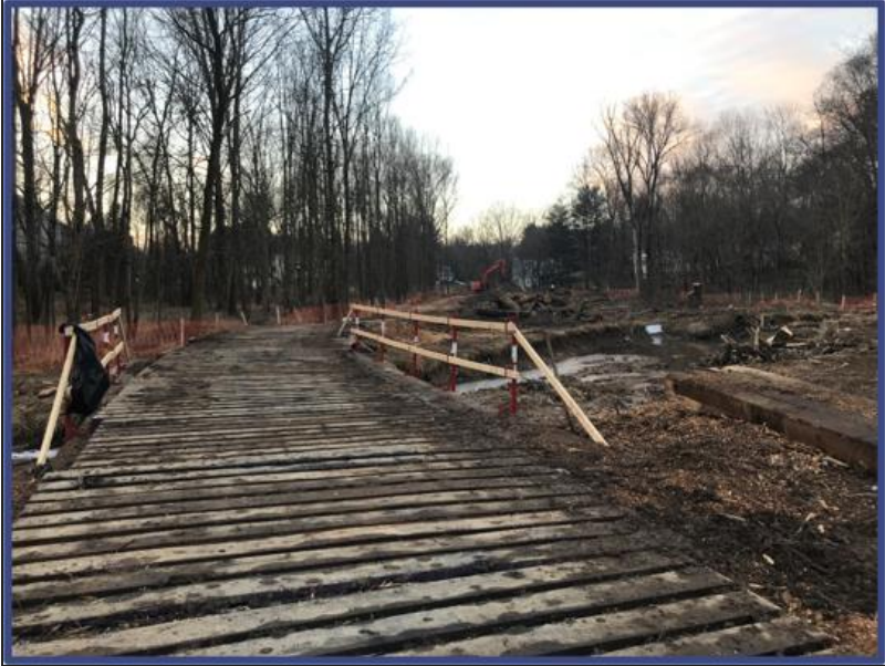
Temporary Stream Crossing
