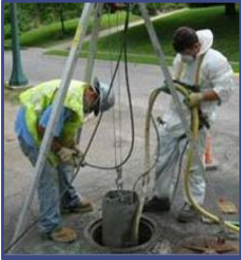
Installing the vent pipe
