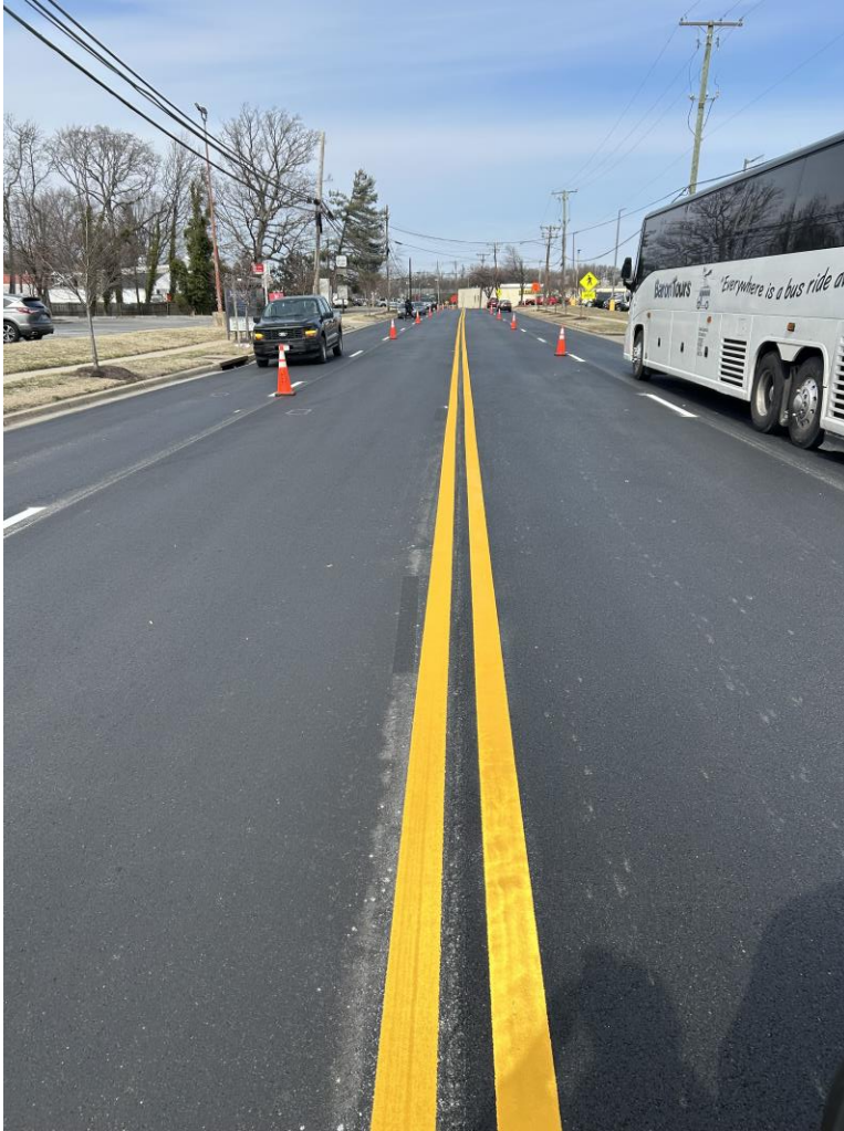
Final paving and striping along Old Branch Ave
