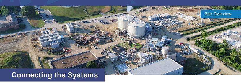
After two years of construction, several major components of the Piscataway Bioenergy project are in place and the staged commissioning of those systems has started. Much of the recent work has been focused on completing the piping and systems that will connect each of the individual process components:
