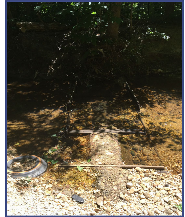
Exposed sewer pipes
