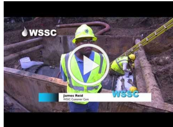
Repairs of a 54" Pipe
