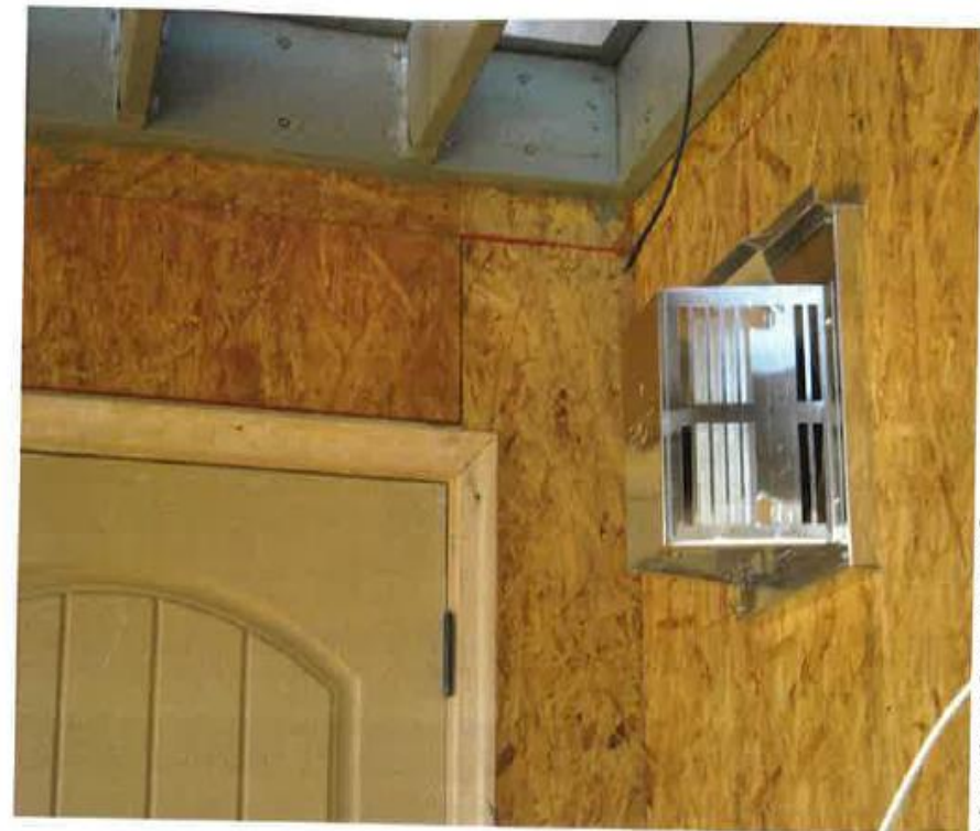
This direct-vent terminal is subject to damage from a swinging door.
