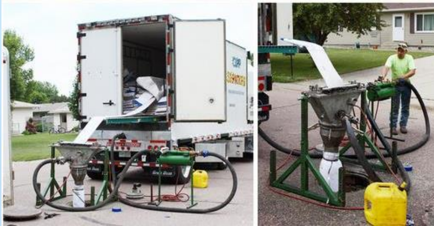
➤ Cured In Place Pipe Reefer Truck
