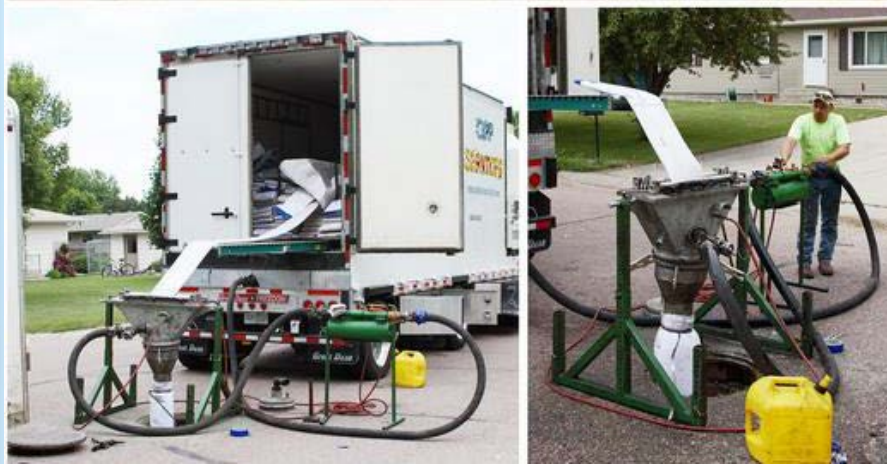
➤ Cured In Place Pipe Reefer Truck
