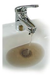
Discolored water contains an accumulation of iron and manganese sediment from rusting cast iron pipes and/or from a buildup of chemical deposits on the pipes. Water steadily flowing at an even pace in one direction will not disturb
