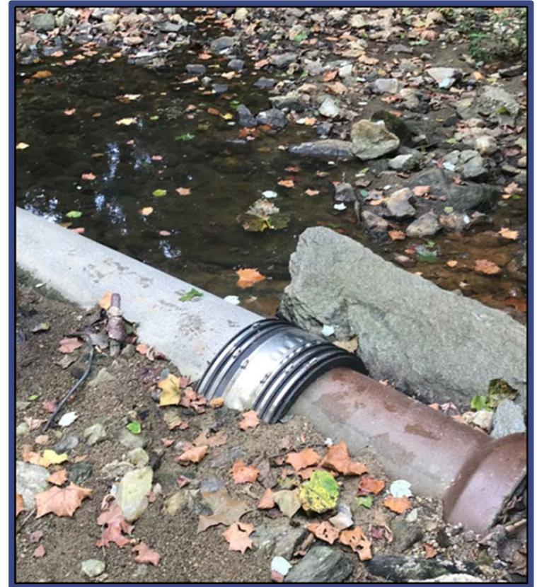
Exposed Sewer in Environmental Sensitive Area
