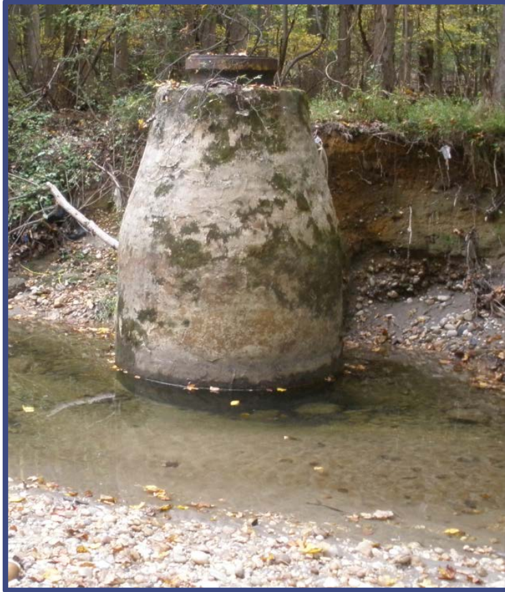
Above-Grade Manhole in Environmental Sensitive Area
