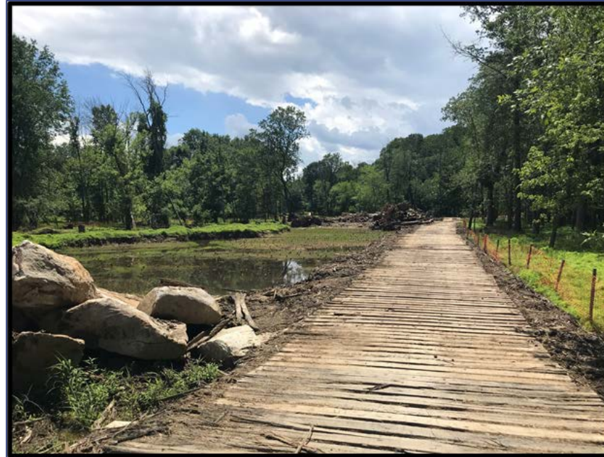
Access Type: Timber Matting
