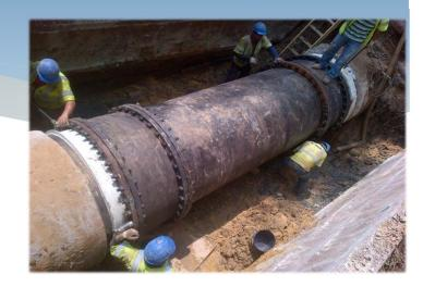
\* For smaller diameters (36" & 42"), dewatering, access, ventilation, etc. may necessitate segment replacement versus CFRP repair
