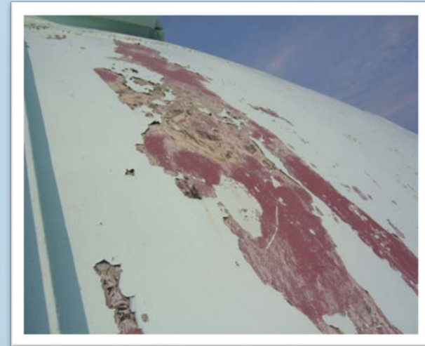
Deteriorating paint on the Camp Springs Water Tank.
