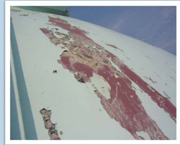
Peeling paint on the side of the tank.
