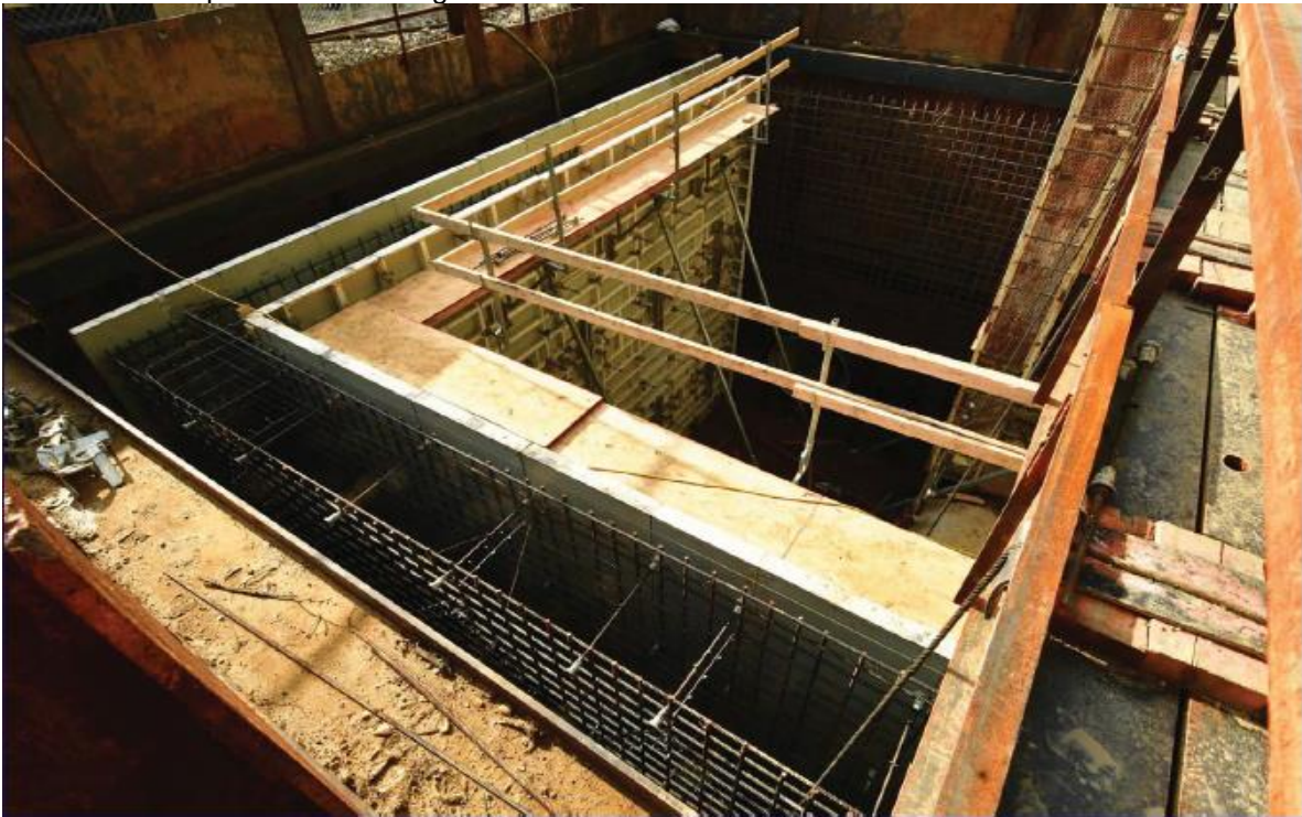
Construction of Transition Structure 2 (TS2) – West side of MD 210 South/Old Fort Road
