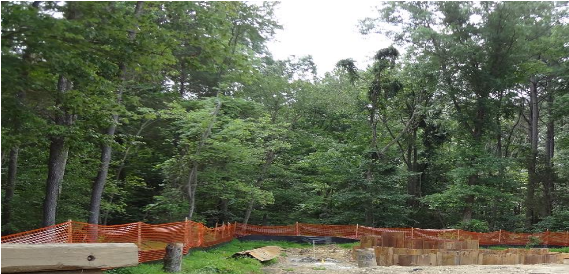
Receiving Shaft location at Broad Creek Pumping Station – Pre excavation
