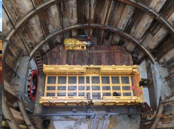
Tunnel launch shaft in front of Harmony Hall
