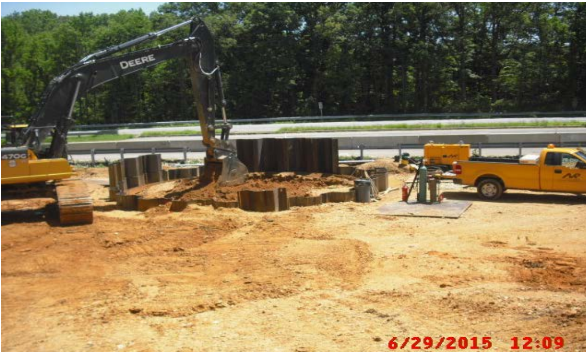
Tunnel Shaft excavation for pipeline along MD 210 - south of Swan Creek Road
