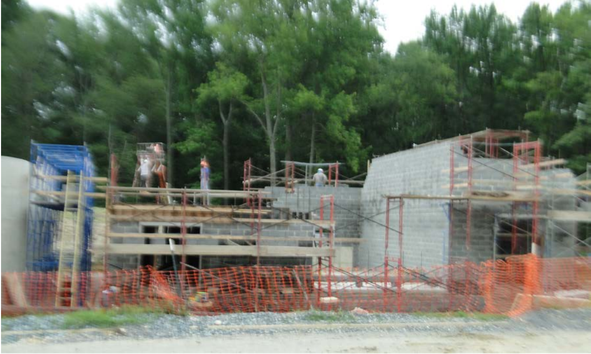
Headworks Facility Construction
