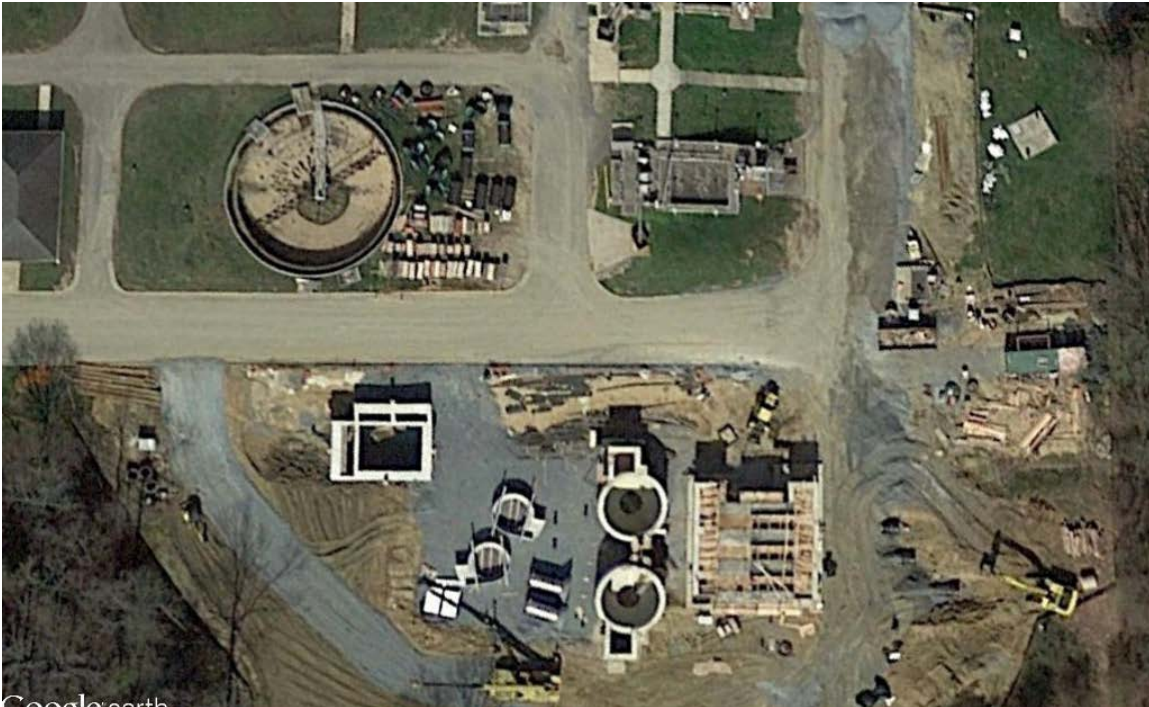
Google Earth Google Earth view of Headworks Facility Construction
