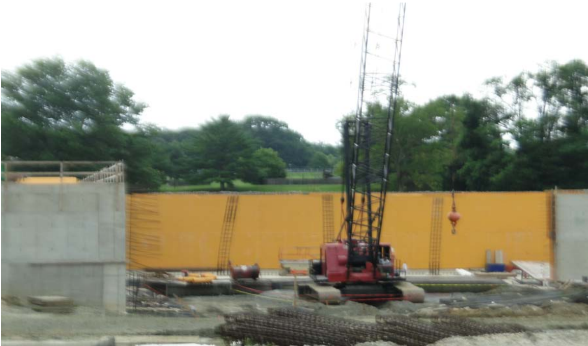
Storage Facility Construction
