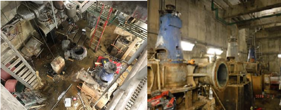
Demolition of existing pumps
