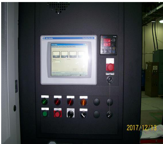
New Variable Frequency Drives (3 vfd's )
