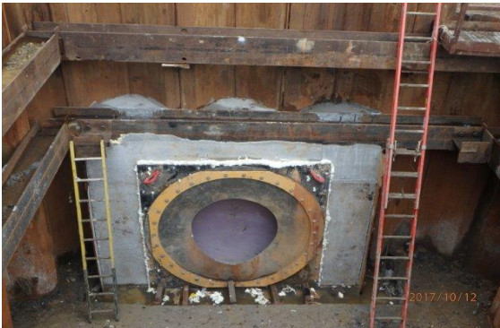
Tunnel Receiving shaft awaits TBM
