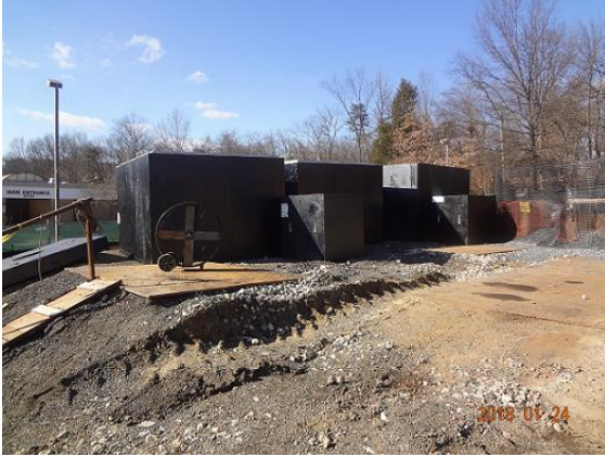
Vaults for MH @ Access Shafts
