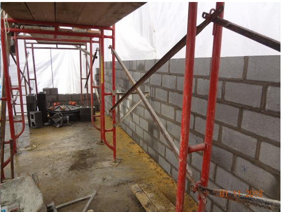
Wall for new electric room @ PS
