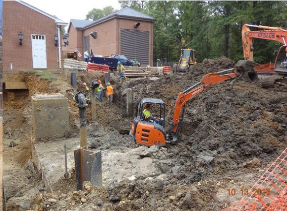
New vault excavation @ PS
