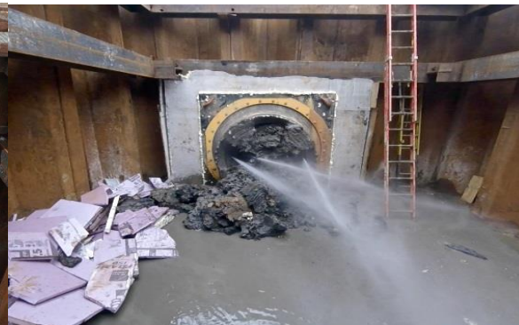
TBM Hole thru – last project tunnel
