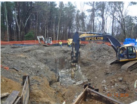
Demolition of existing 36" FM @ PS
