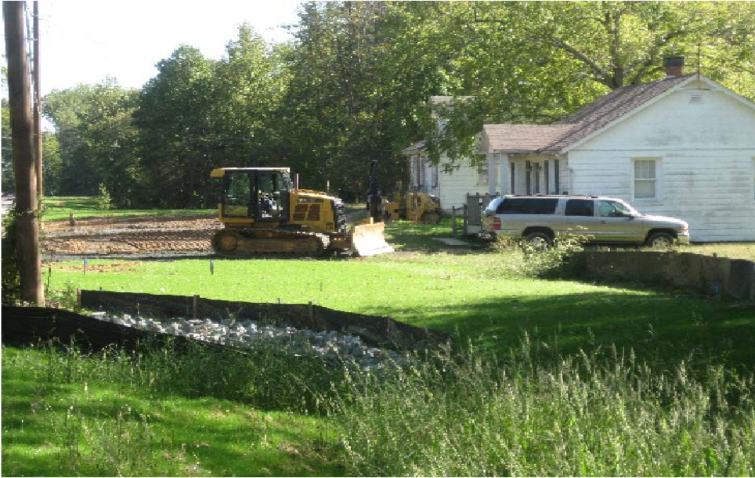
Site Restoration work along Livingston Road between Fort Washington Road and Cornett Street
