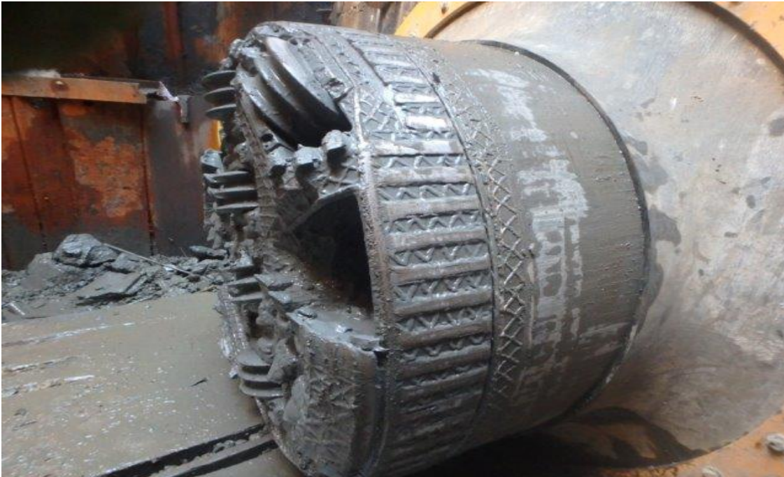
Hole thru of Micro Tunnel Boring Machine on Tunnel 7 (From Piscataway Plant across Piscataway Creek)
