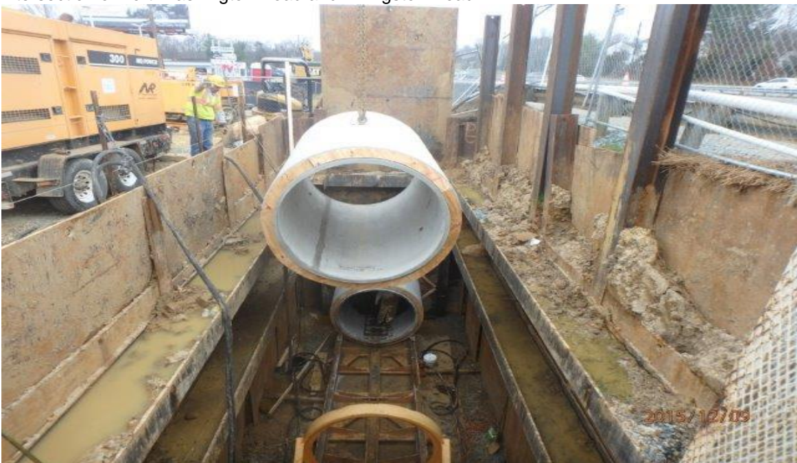
Casing pipe installation along MD 210 at Cornett Street for new force main
