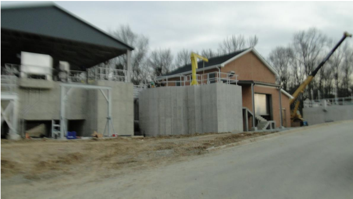
Headworks Facility Construction
