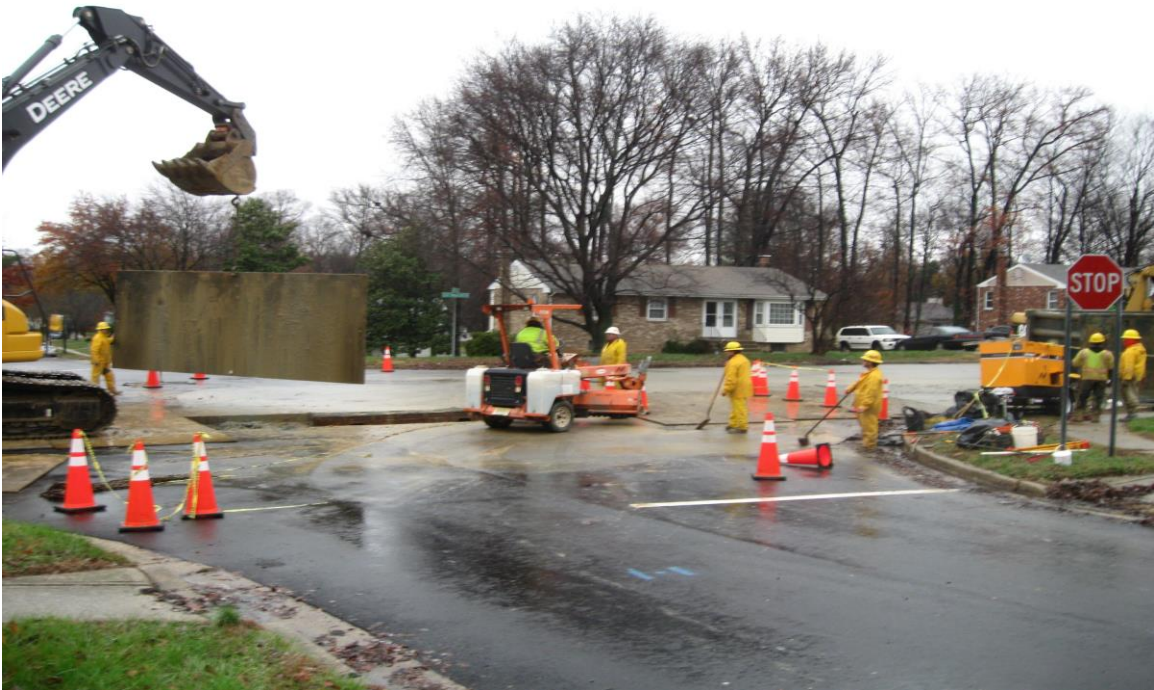
Pipeline Construction along Tantallon Drive for connection to Swan Creek WWPS force main
