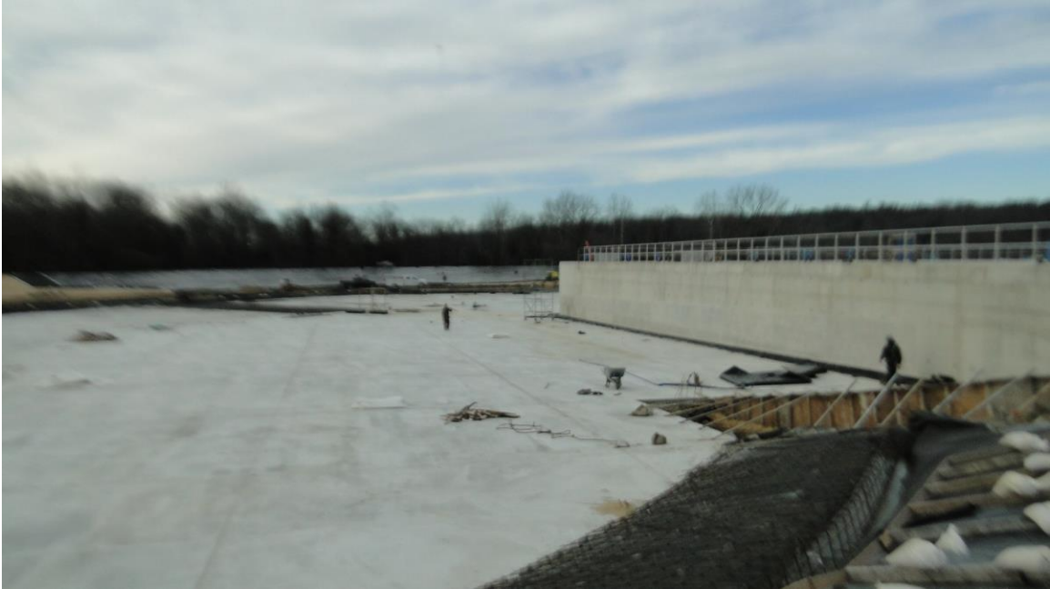
Storage Facility Construction
