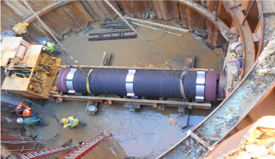
Installation of 48" carrier pipe for new force main along MD 210 – south of Old Fort Road
