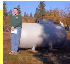
600 Gal Propane Tank
