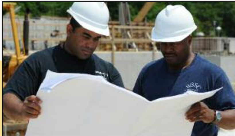
WSSC workers at the Parkway Wastewater Treatment Plant.
