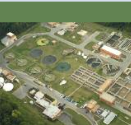
Parkway Wastewater Treatment Plant
