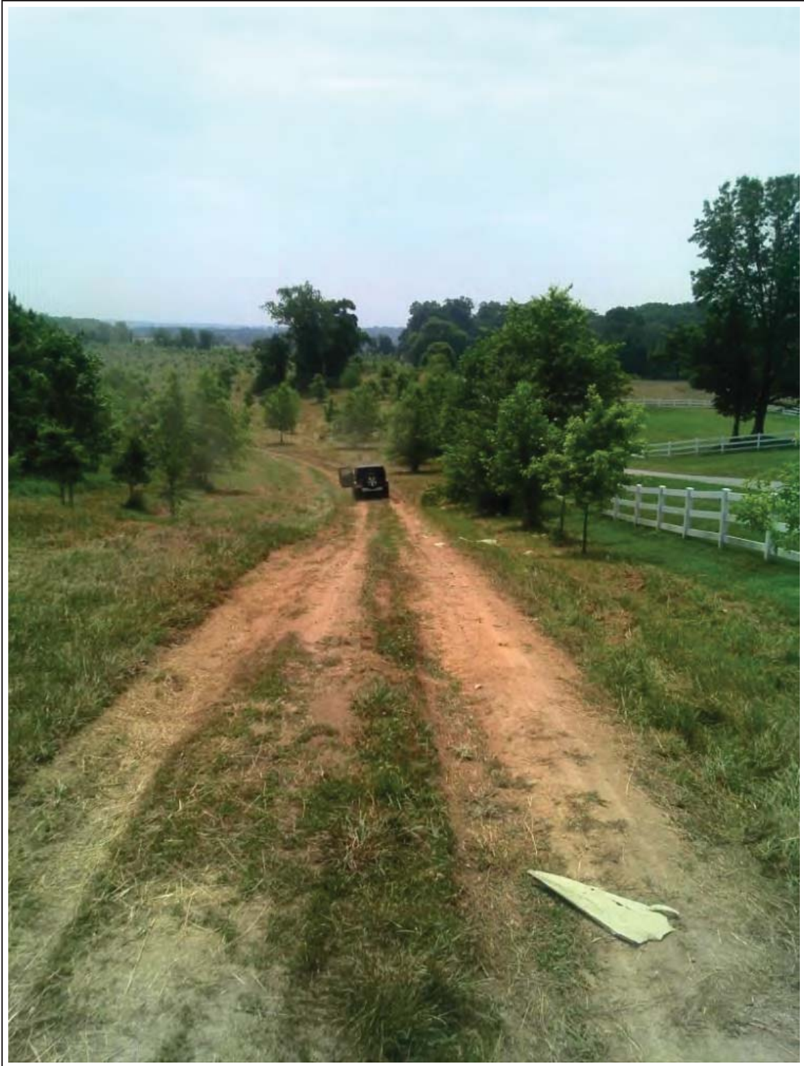
Photo 5-39: Triadelphia Lake Road rutting from vehicles
