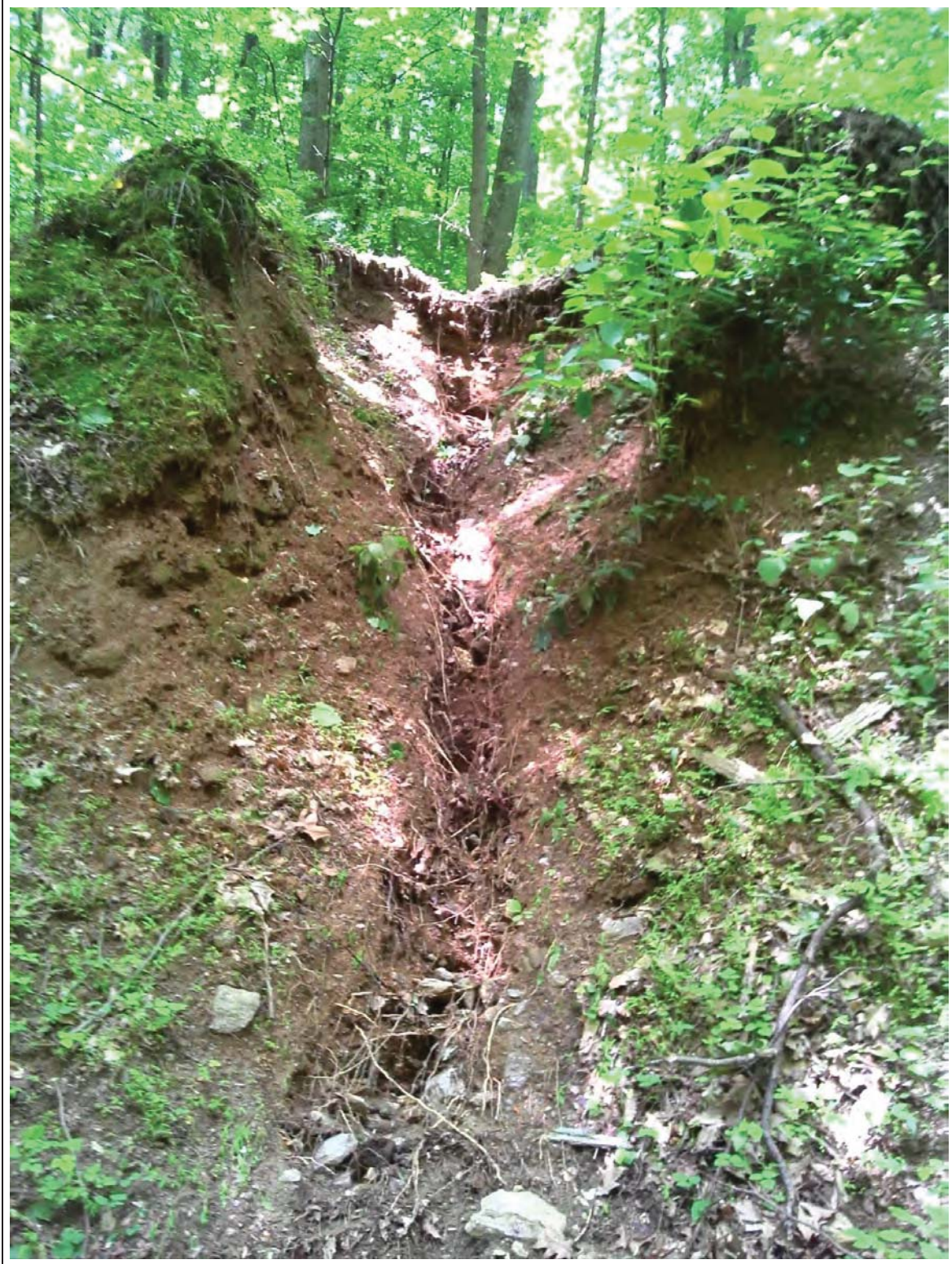
Photo 5-25: Washout area within Section 5 of the Access Road
