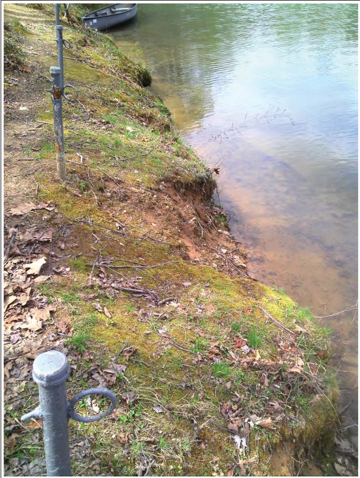
Photo 5-78: Greenbridge Recreational Area bank erosion with un-stabilized slopes
