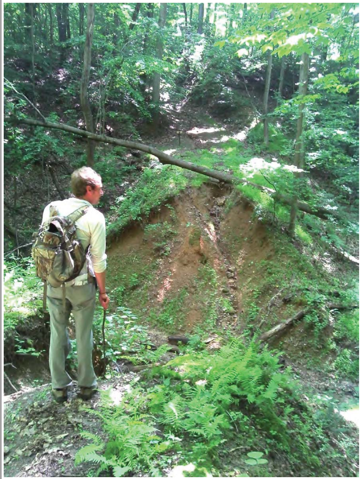
Photo 5-24: Washout area within Section 5 of the Access Road
