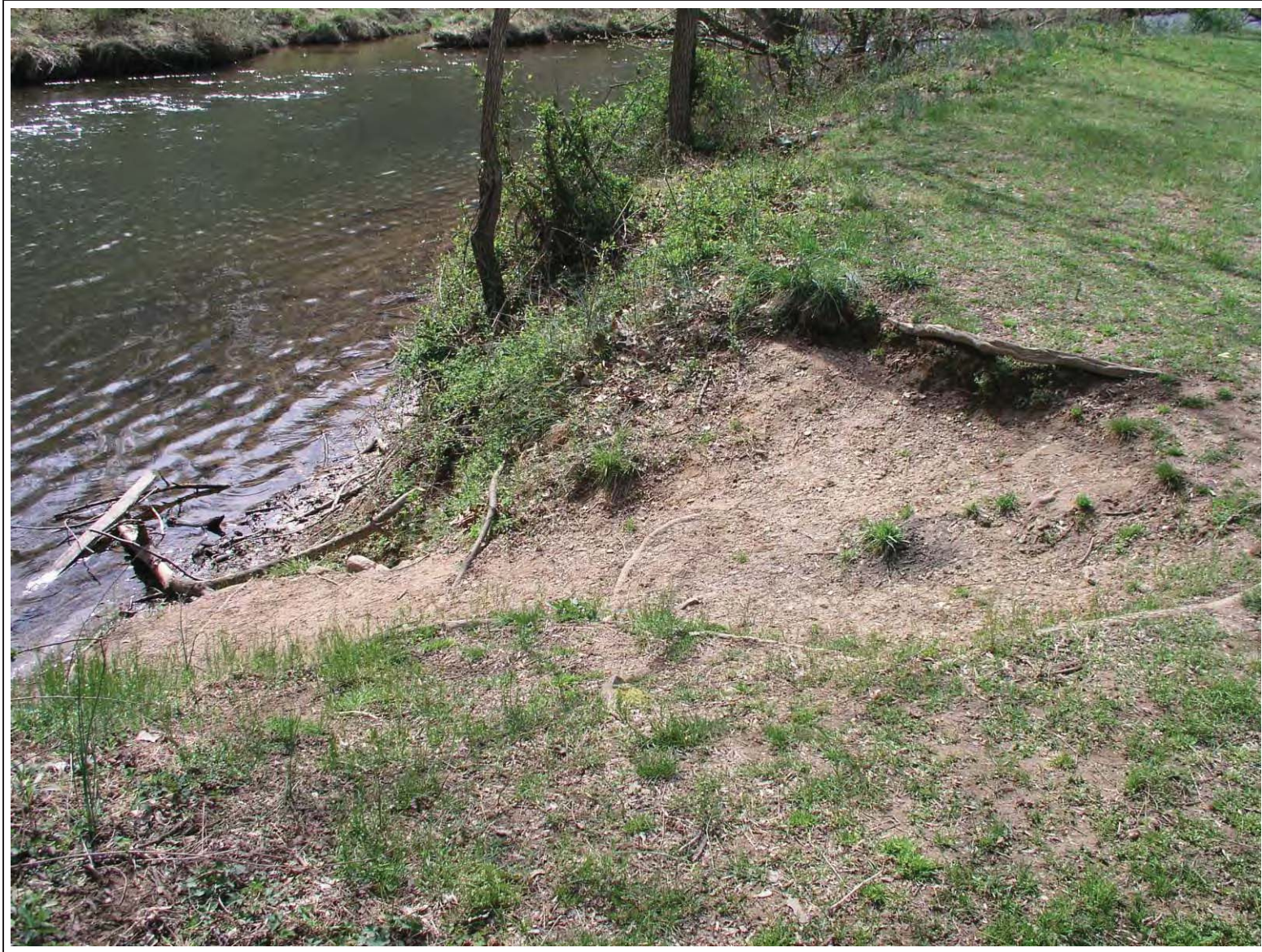
Photo 5-66: Brighton Dam localized bank erosion due to fishing access to edge of water
