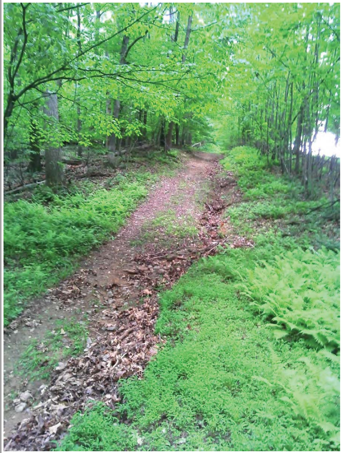
Photo 5-21: Pat Oliva Trail channelized erosion
