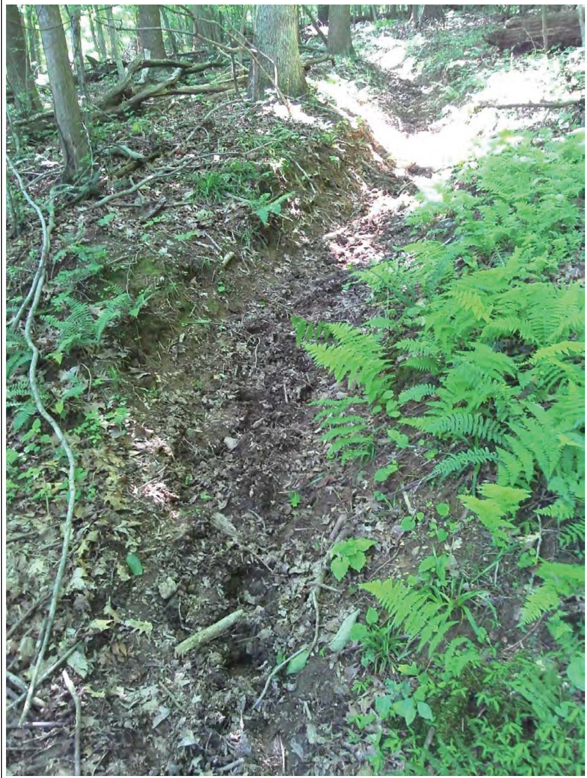
Photo 5-20: Pat Oliva Trail channelized erosion
