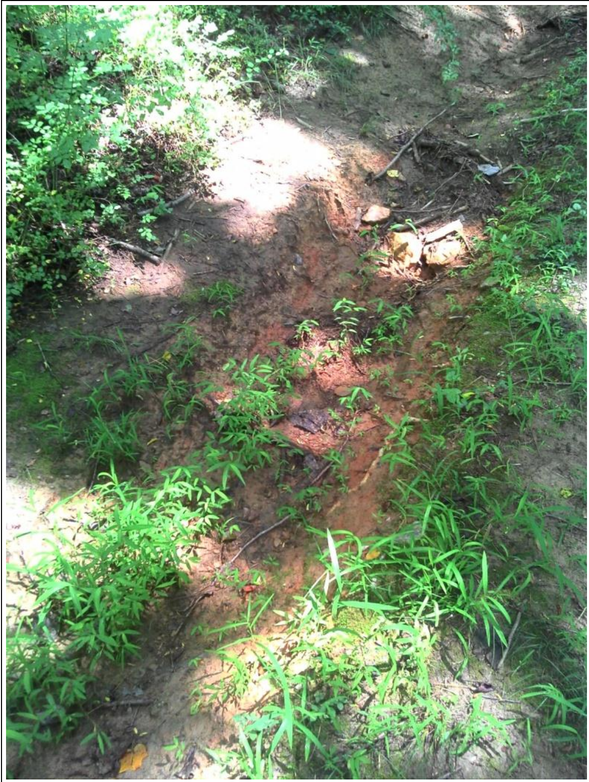
Photo 5-42: Greenbridge West Access Rd significant rutting and erosion
