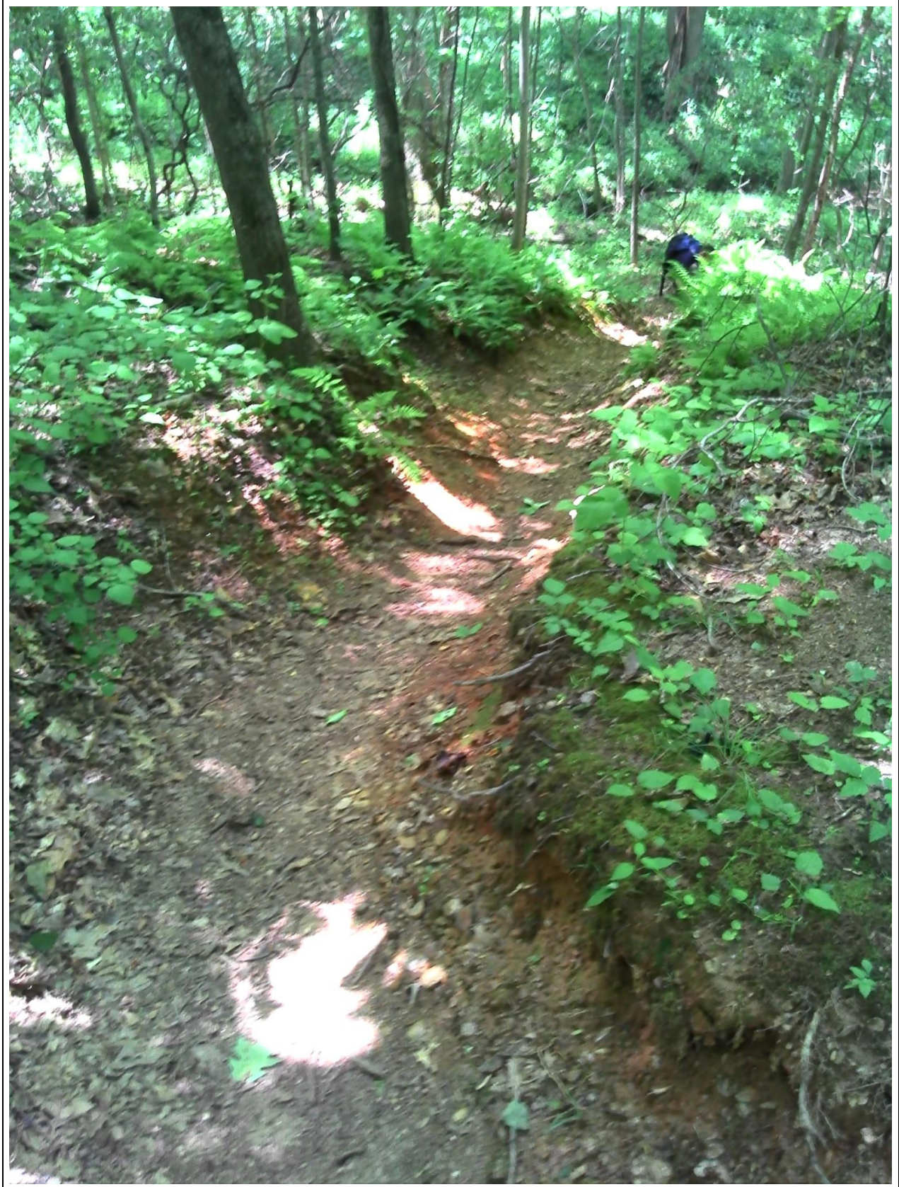
Photo 5-19: Pat Oliva Trail section eroded due to poor trail alignment
