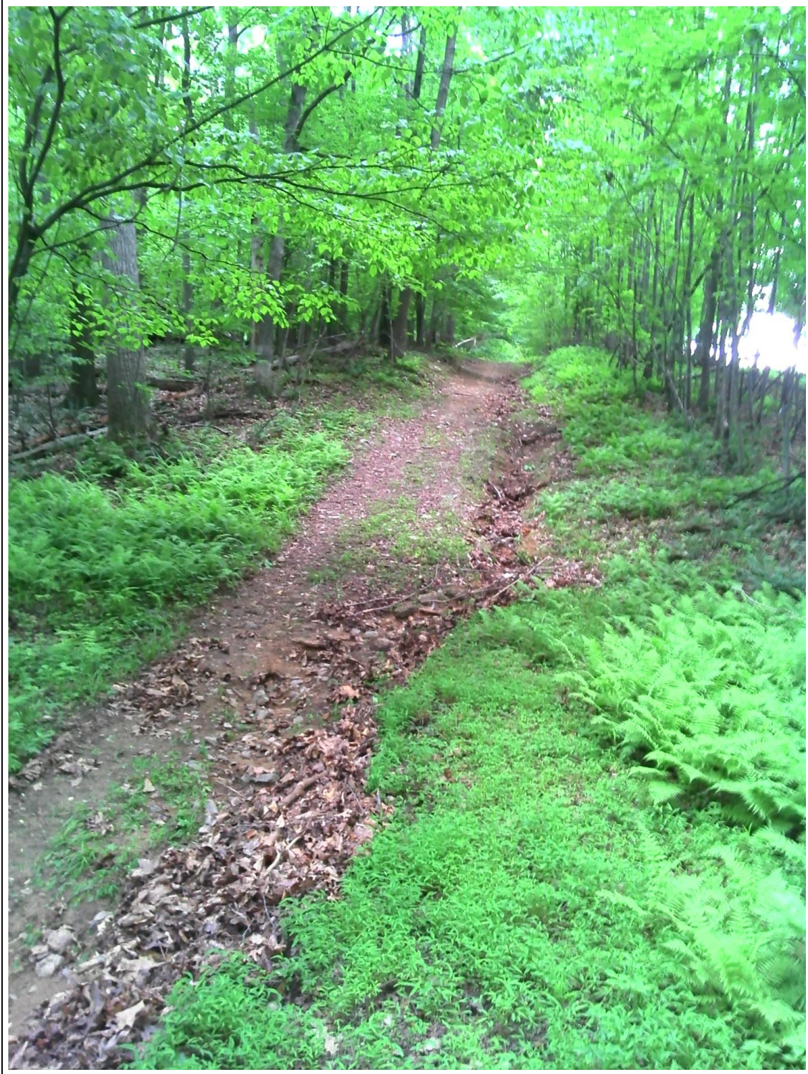
Photo 5-21: Pat Oliva Trail channelized erosion
