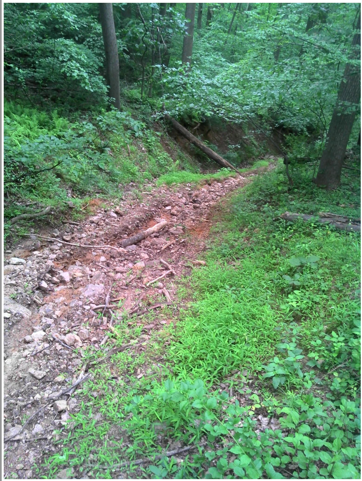
Photo 7: Section 2 typical steep hill with erosion and rock footing.
