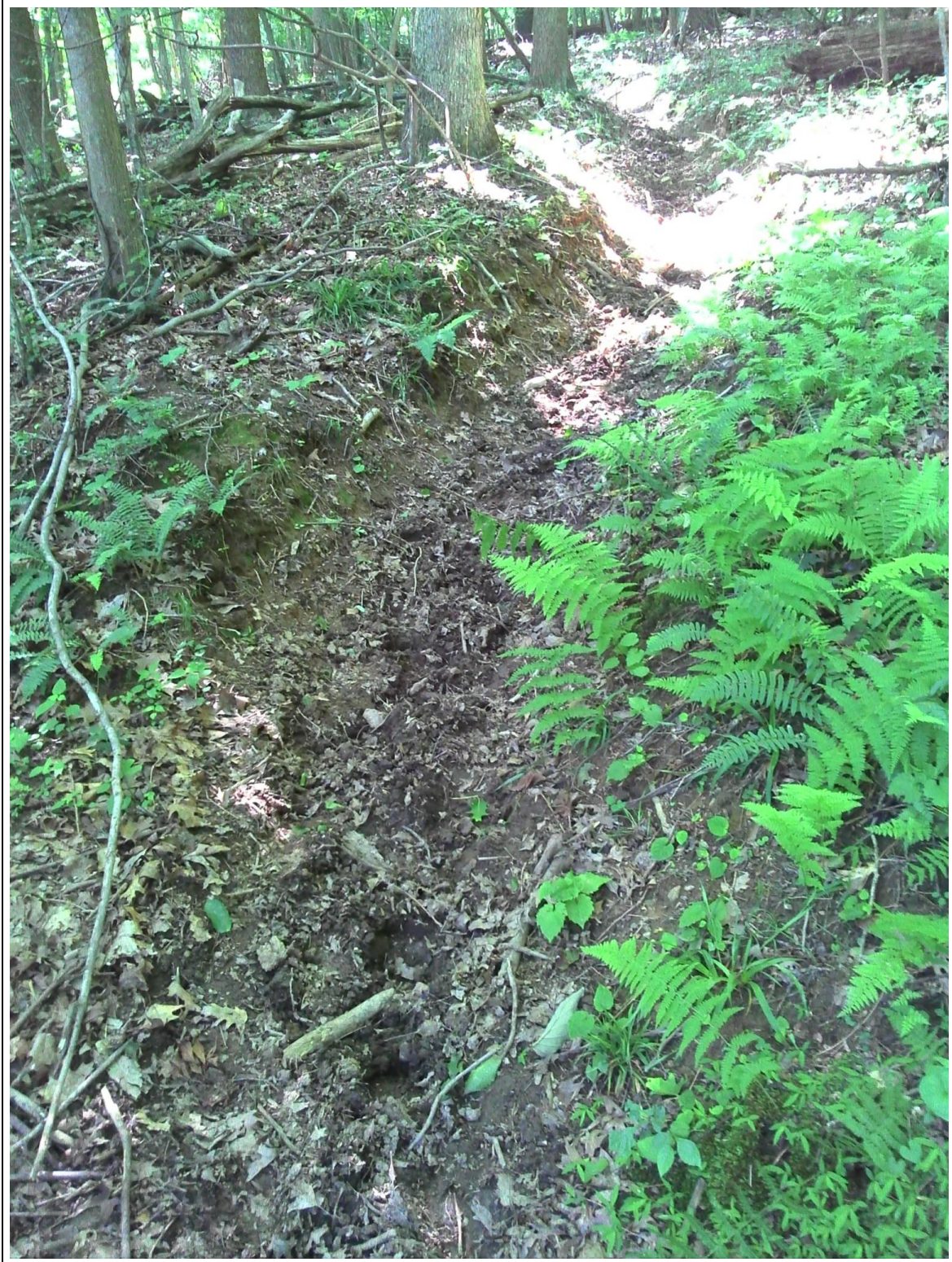
Photo 5-20: Pat Oliva Trail channelized erosion
