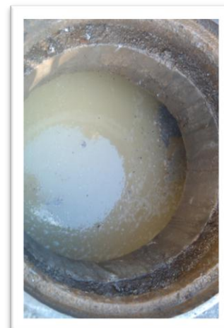
Figure 3.10. Ice Cream Shop's GAD, 2 nd Chamber, showing greater accumulation towards interceptor walls - 1/14/11
