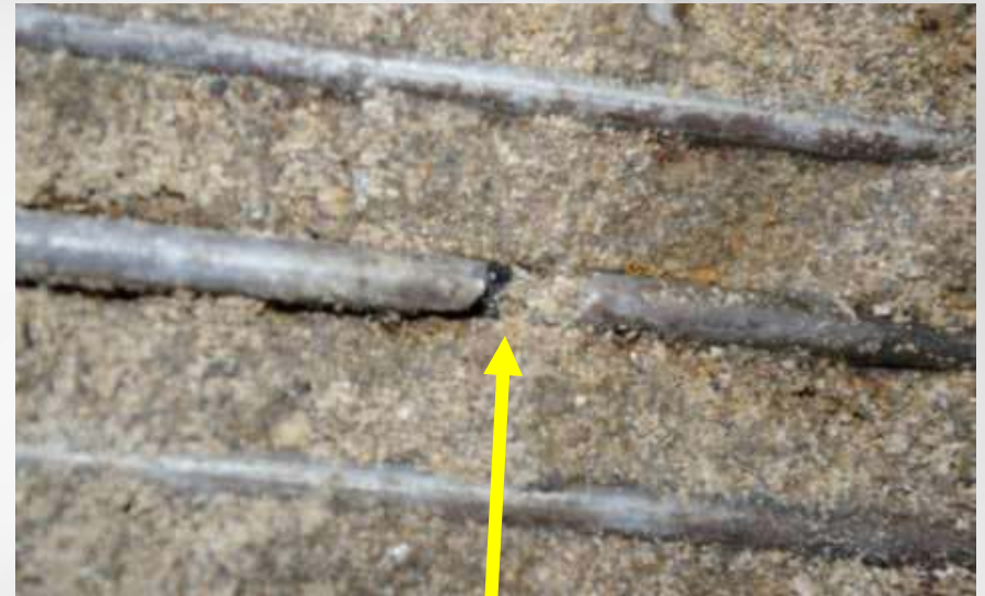
Wire Tensile Fracture
