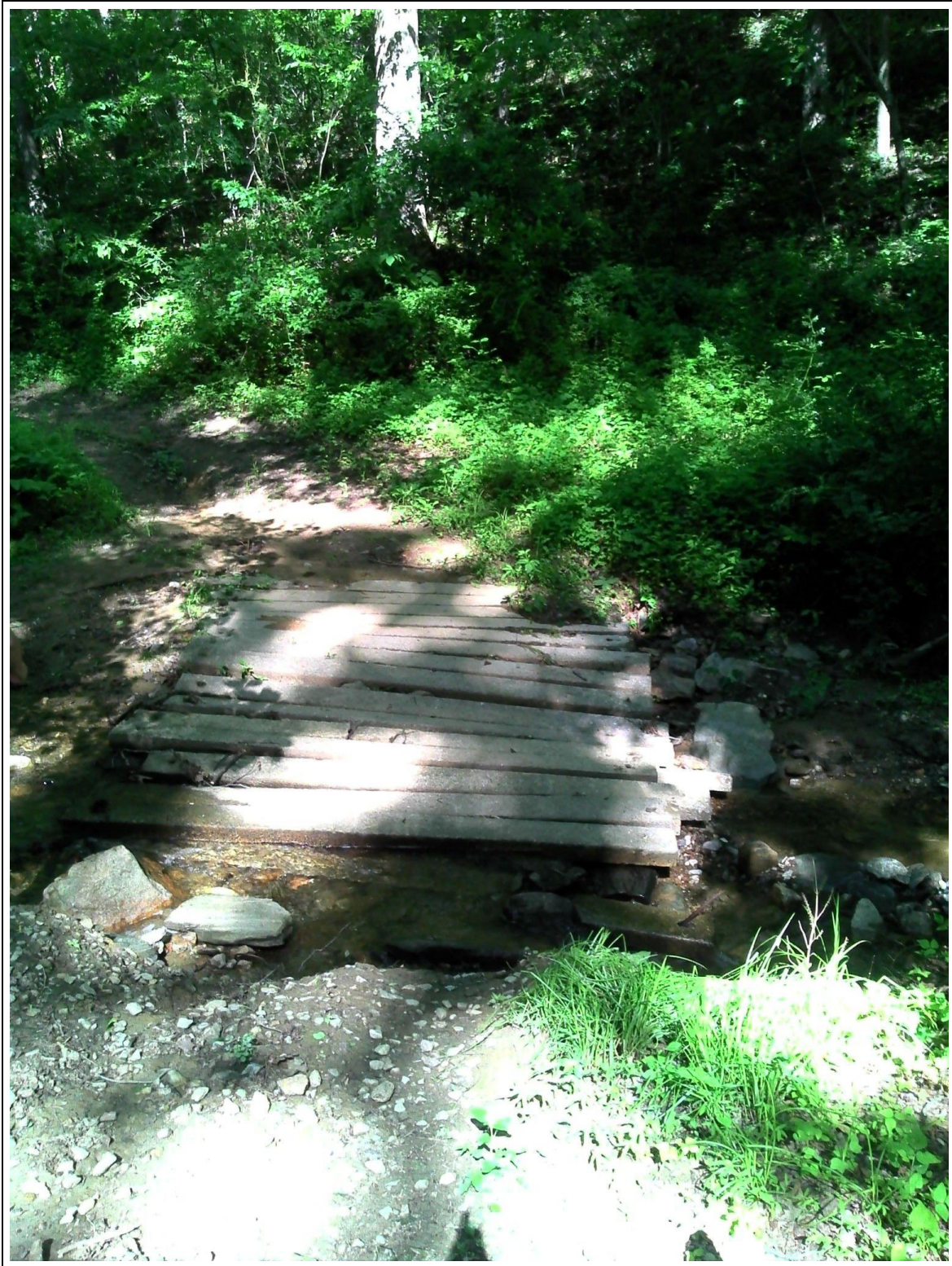
Photo 4: Section 1 stream crossing with washed out railroad ties
