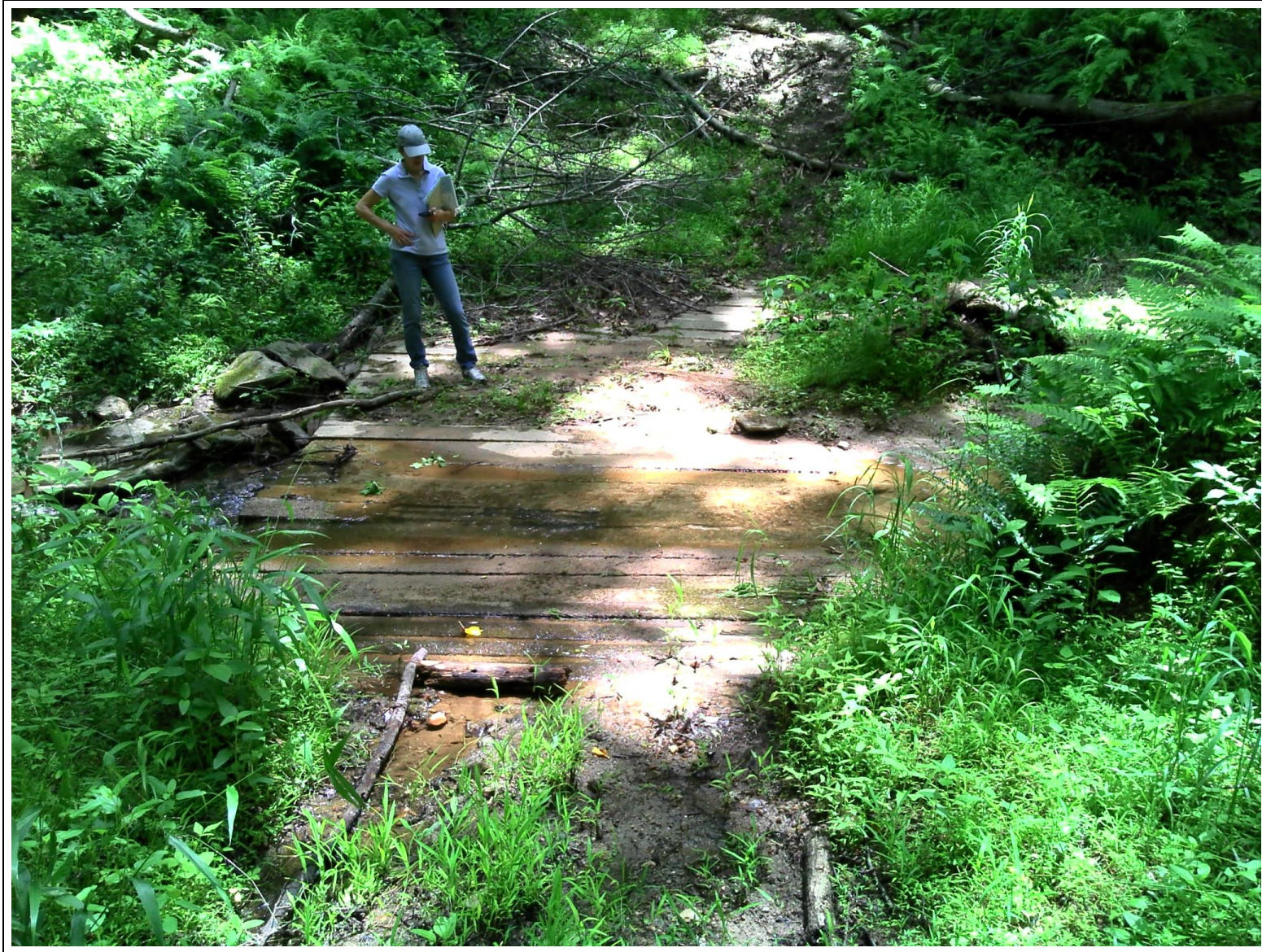
Photo 13: Section 4 stream crossing with railroad ties/rebar.
