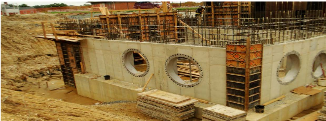
Headworks Facility Construction
