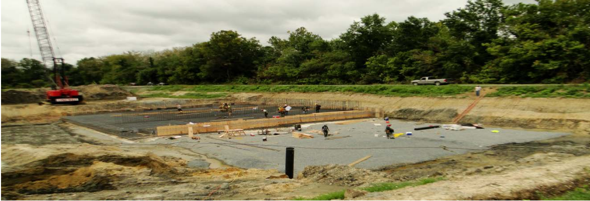
Storage Facility Construction – Base slab
