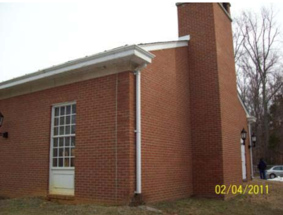
Existing South Elevation from Southwest corner
