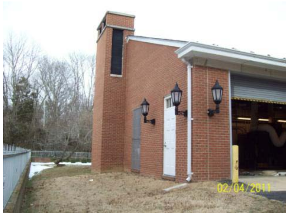
Existing South Elevation from Southeast corner
