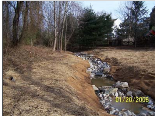
Cherry Creek Stream Construction
