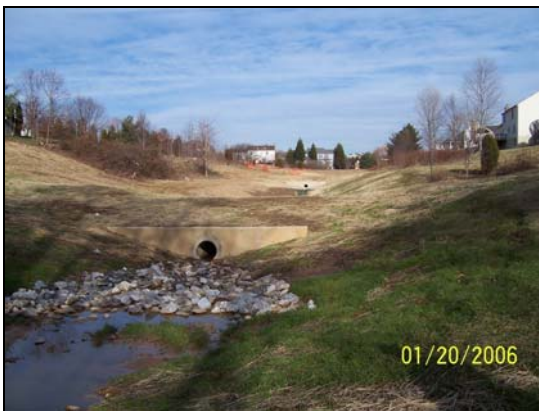
Cherry Creek Ponds Construction
