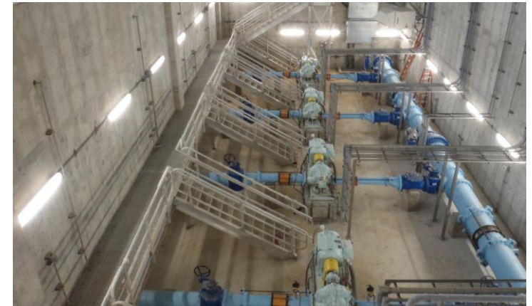
Brink Zone Reliability Improvements
