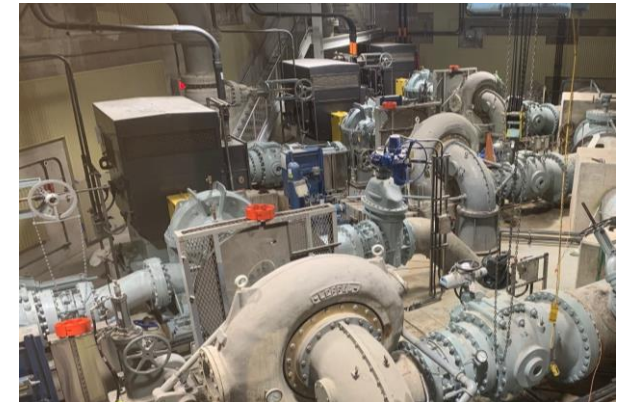
Rocky Gorge Pump Station
