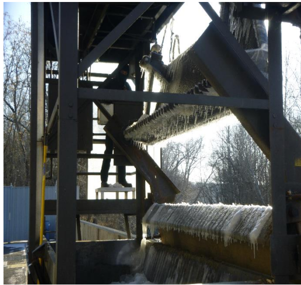
Trash rake used around the clock at Potomac WFP to remove ice from intake bar screens
