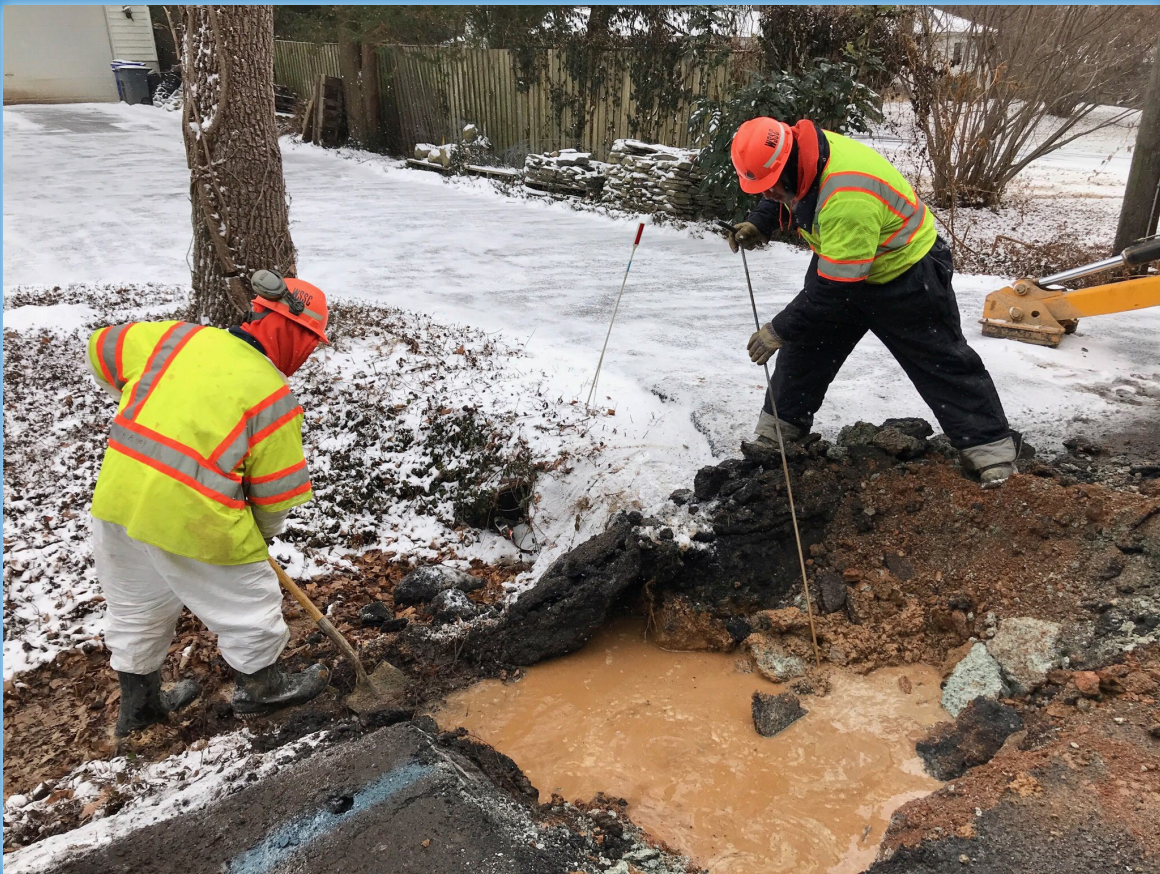
Lyttonsville Crew Working on Water Main Break January 2018
